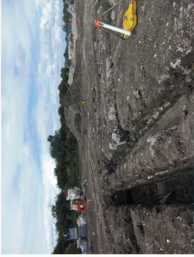
Plate 34. View of House Footings. Facing North-west.
