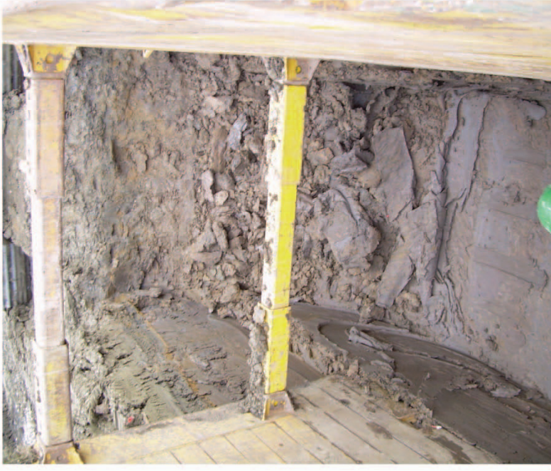
Plate 16. View of the Excavation of Drainage Trenches, Facing East.
