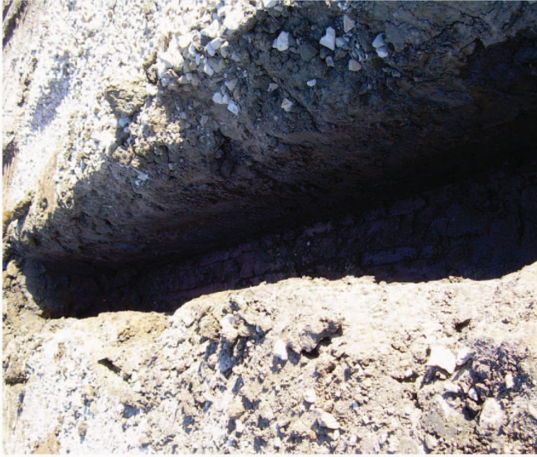
Plate 23. View of the Excavation of Drainage Trenches, Facing South.
