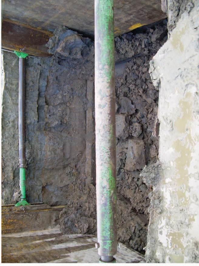
Plate 10. View of the Excavation of Drainage Trenches, Facing East.
