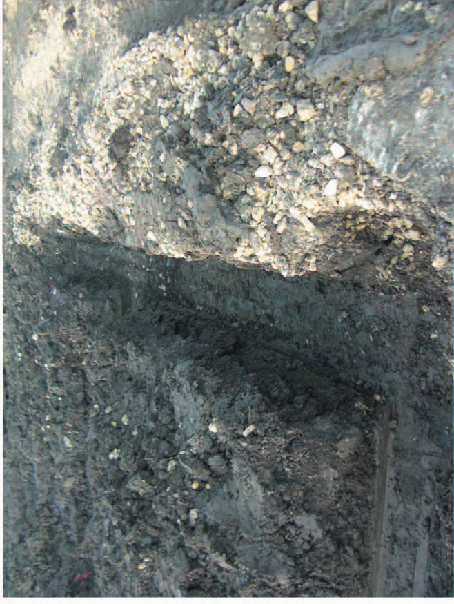
Plate 42. View of House Footings. Facing West.
