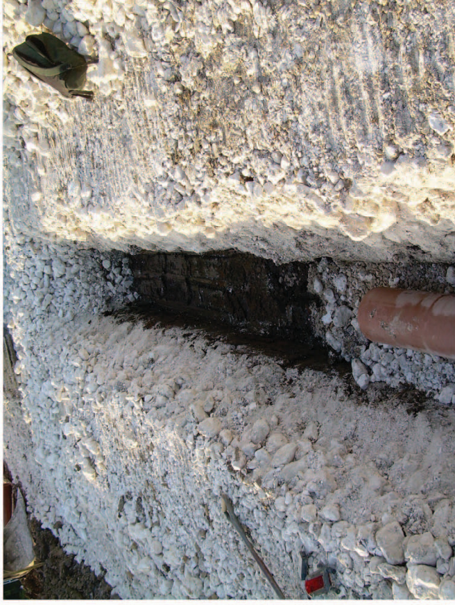
Plate 18. View of the Excavation of Drainage Trenches, Facing South.
