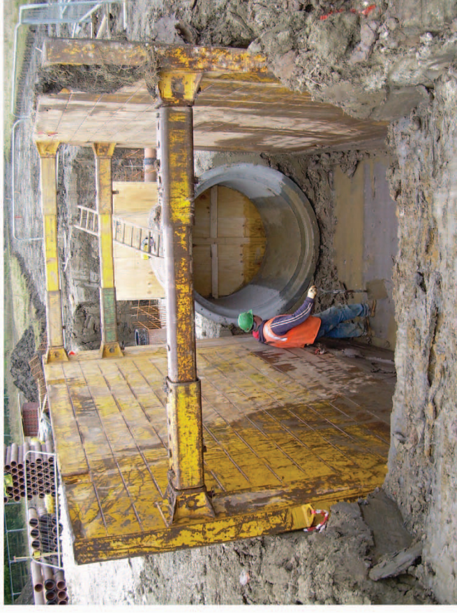
Plate 14. View of the Excavation of Drainage Trenches, Facing East.
