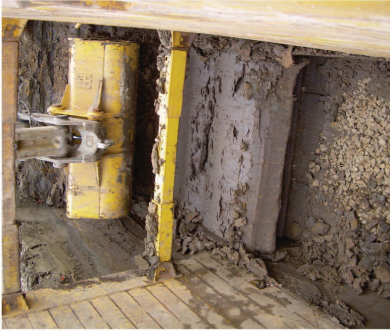
Plate 15. View of the Excavation of Drainage Trenches, Facing East.
