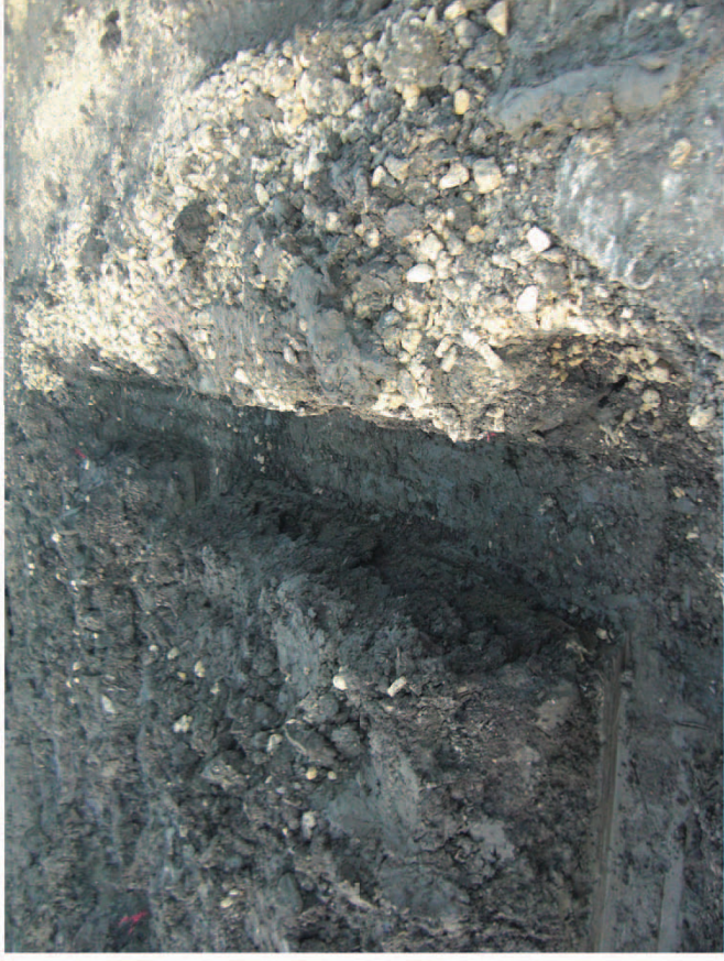
Plate 42. View of House Footings. Facing West.
