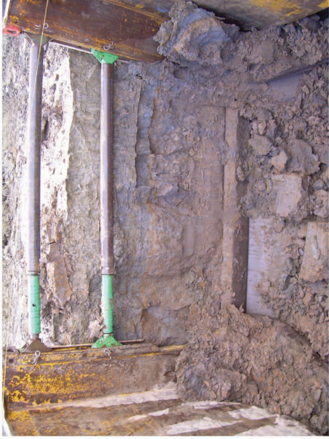
Plate 11. View of the Excavation of Drainage Trenches, Facing East.
