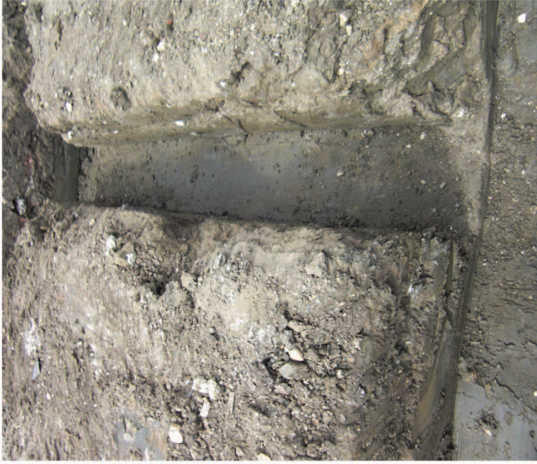
Plate 37. View of House Footings. Facing West.
