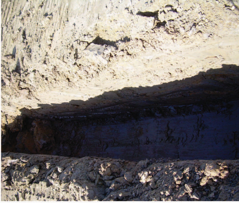
Plate 21. View of the Excavation of Drainage Trenches, Facing South.
