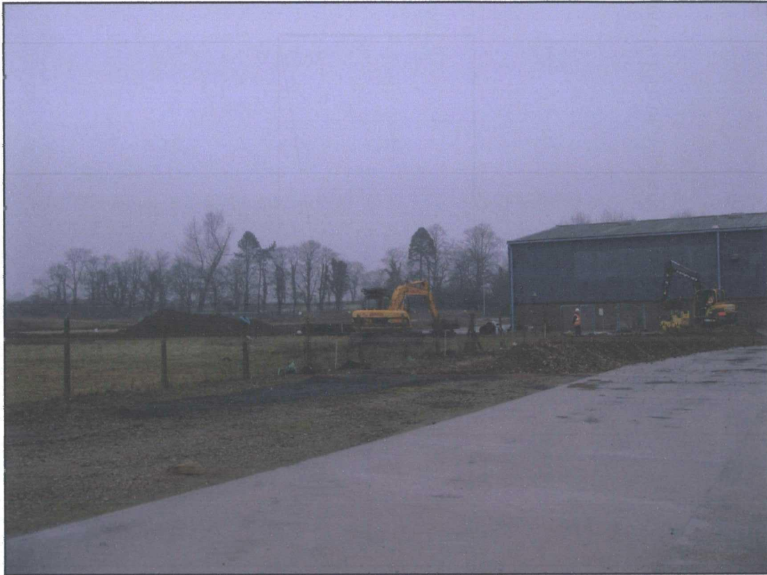
Plate 1. General view to north-east of stockpile area during works.
