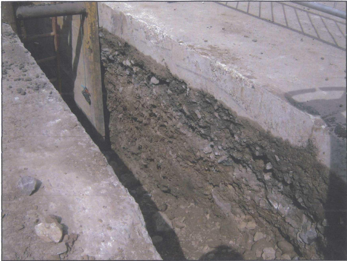
Plate 5. General view of excavation of service trench.
