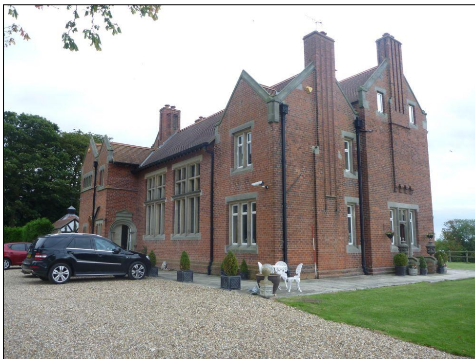
Plate 10 The south-west and north-west facades of the hall, looking north-east
