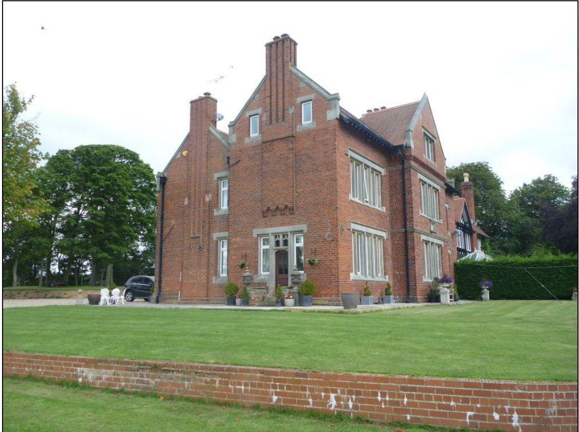
Plate 9 The south-west and south-east facades of the hall, looking north
