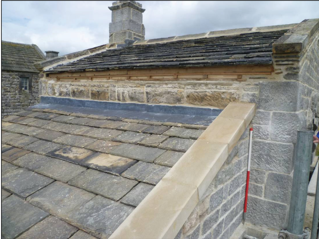
Plate 7: New roof pitch to south cell, with bat-friendly fascia, looking N (photo 3/093).
