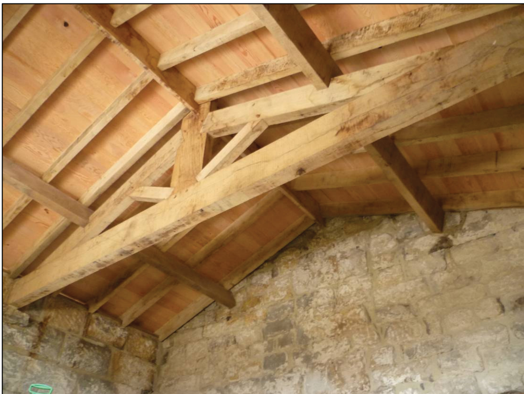
Plate 6: New roof truss to central cell, looking N (photo 3/089).
