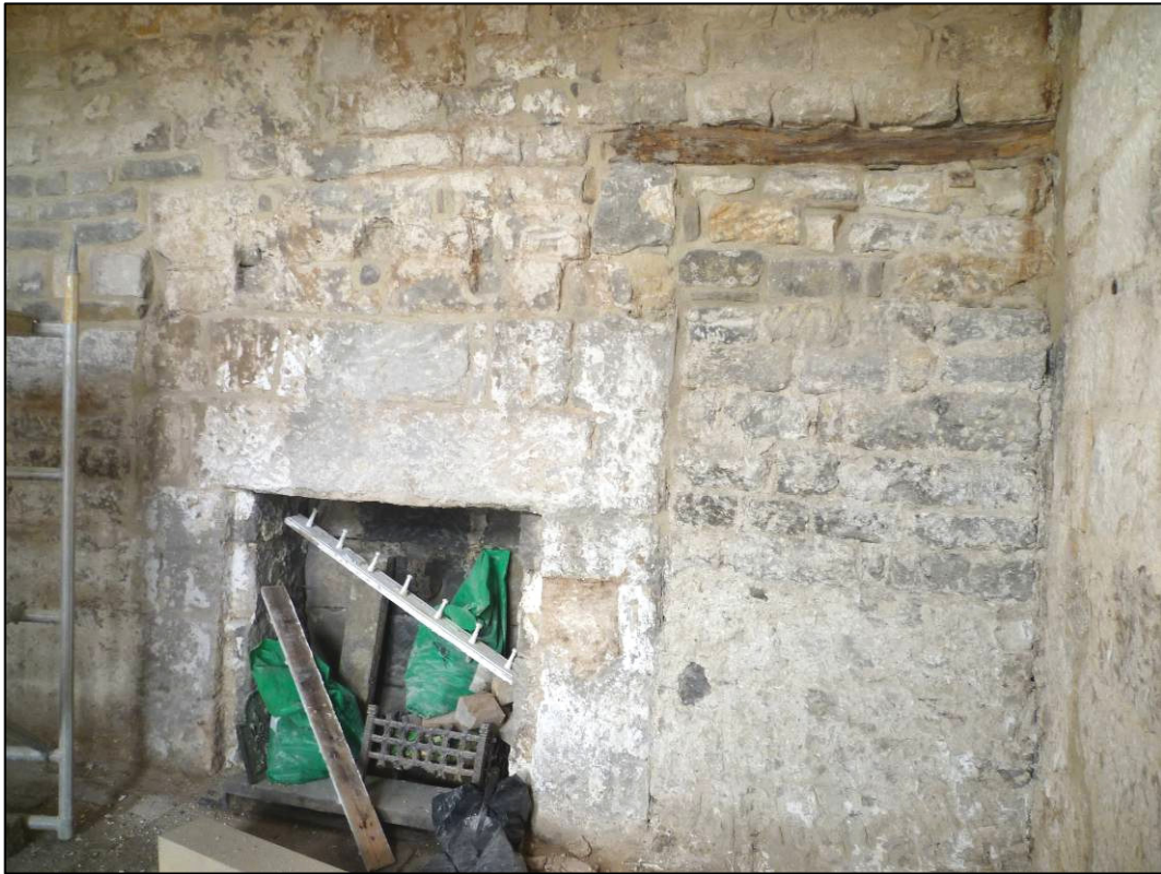
Plate 5: North end of central cell after removal of plaster, showing blocked niche and recesses over fireplace, looking W (photo 3/087).
