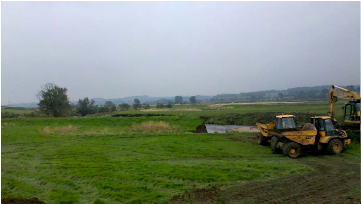
Plate 3: Embankment 105 , looking south-west
