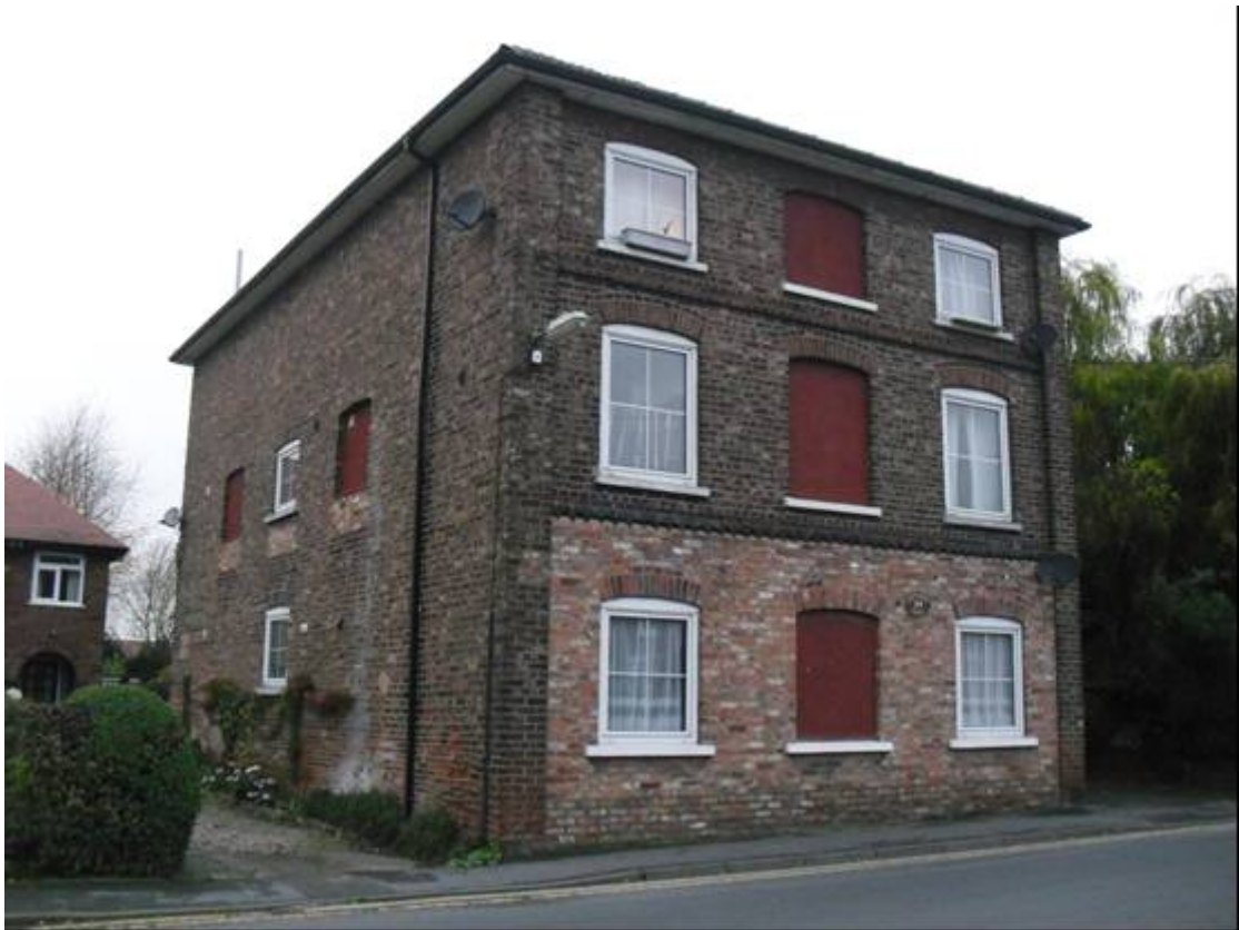
Plate 20 Former warehouse or workshop, No 39 Main Street, looking west
