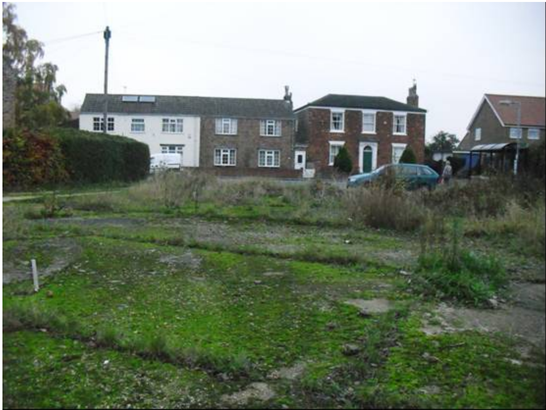
Plate 5 Looking back towards Main Street towards farm Gaz No 7 (left) and former chapel Gaz No 8 (right)
