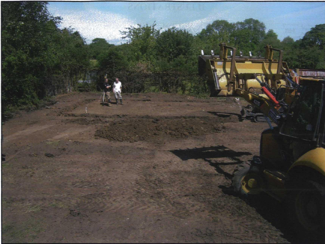
Plate 1. General shot of site of garage during ground works, looking north.
