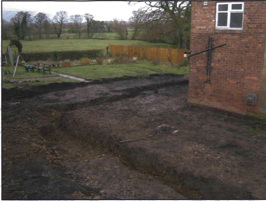
Plate 3. General view of foundations trench for extension, looking north-east.
