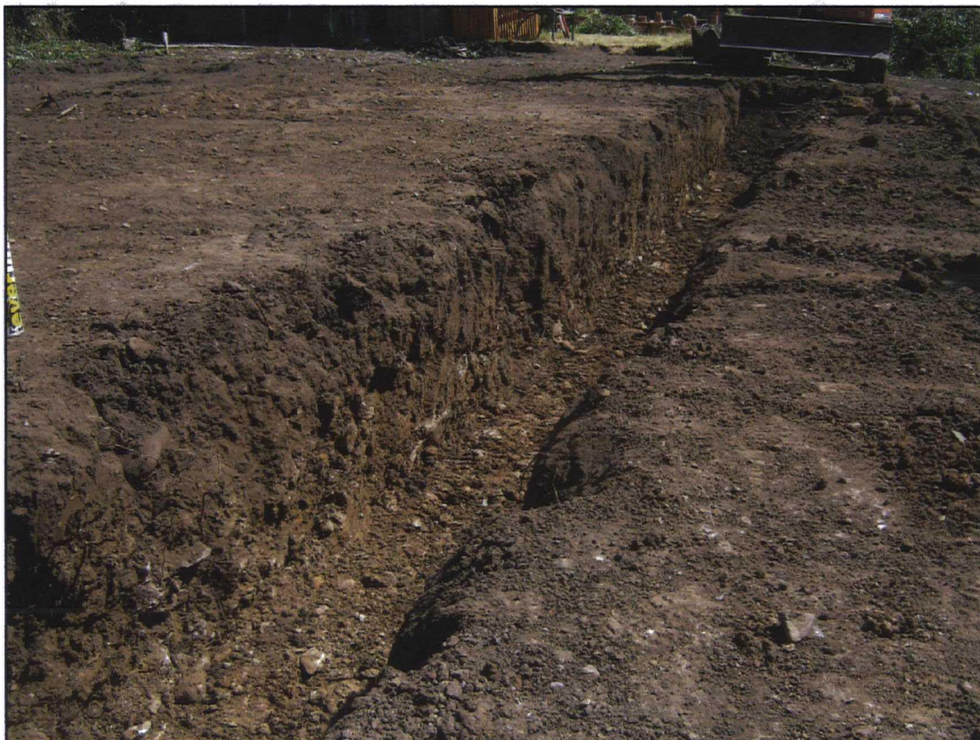
Plate 2. General view of foundations trench for garage, looking north-east.
