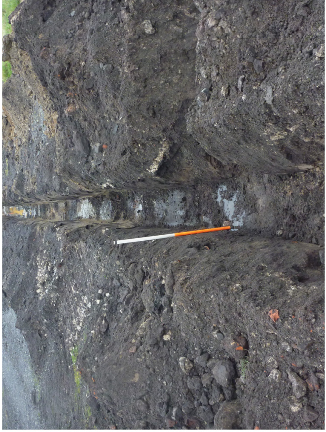
Plate 5. Southern Section of Cable Trench after Excavation Facing South.
