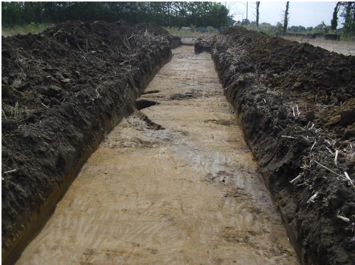
Plate 8: Trench 6 – looking south (1m scale)
