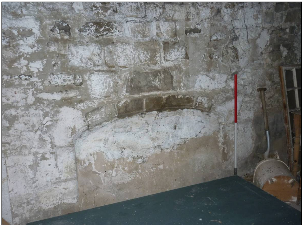
Plate 7: Medieval building, first floor blocked fireplace in east wall, looking SE (photo 3/865).
