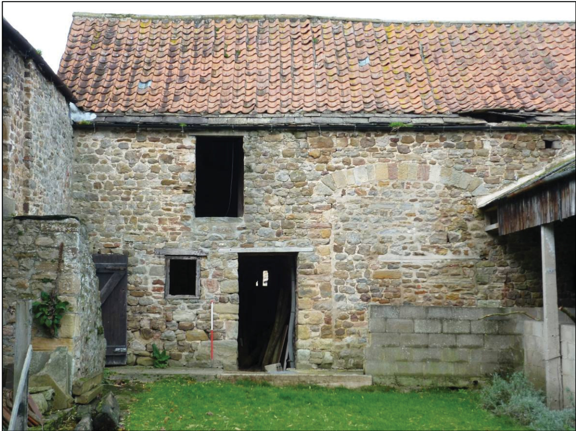
Plate 10: Barn, west end of south elevation, looking N (photo 1/535).
