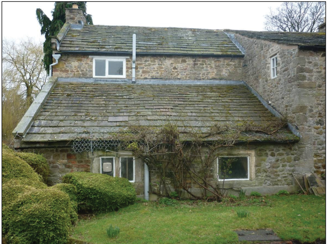
Plate 15: Hall, north elevation of outshut, looking S (photo 4/836).
