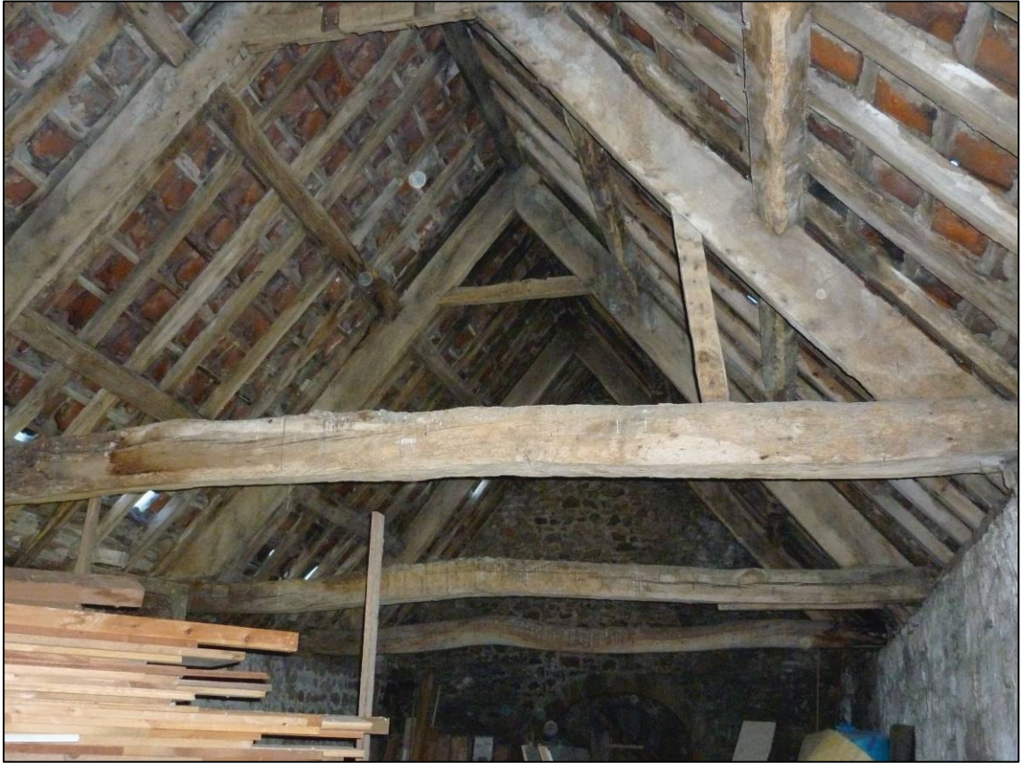
Plate 8: Medieval building, first floor truss ('III'), looking N (photo 3/866).
