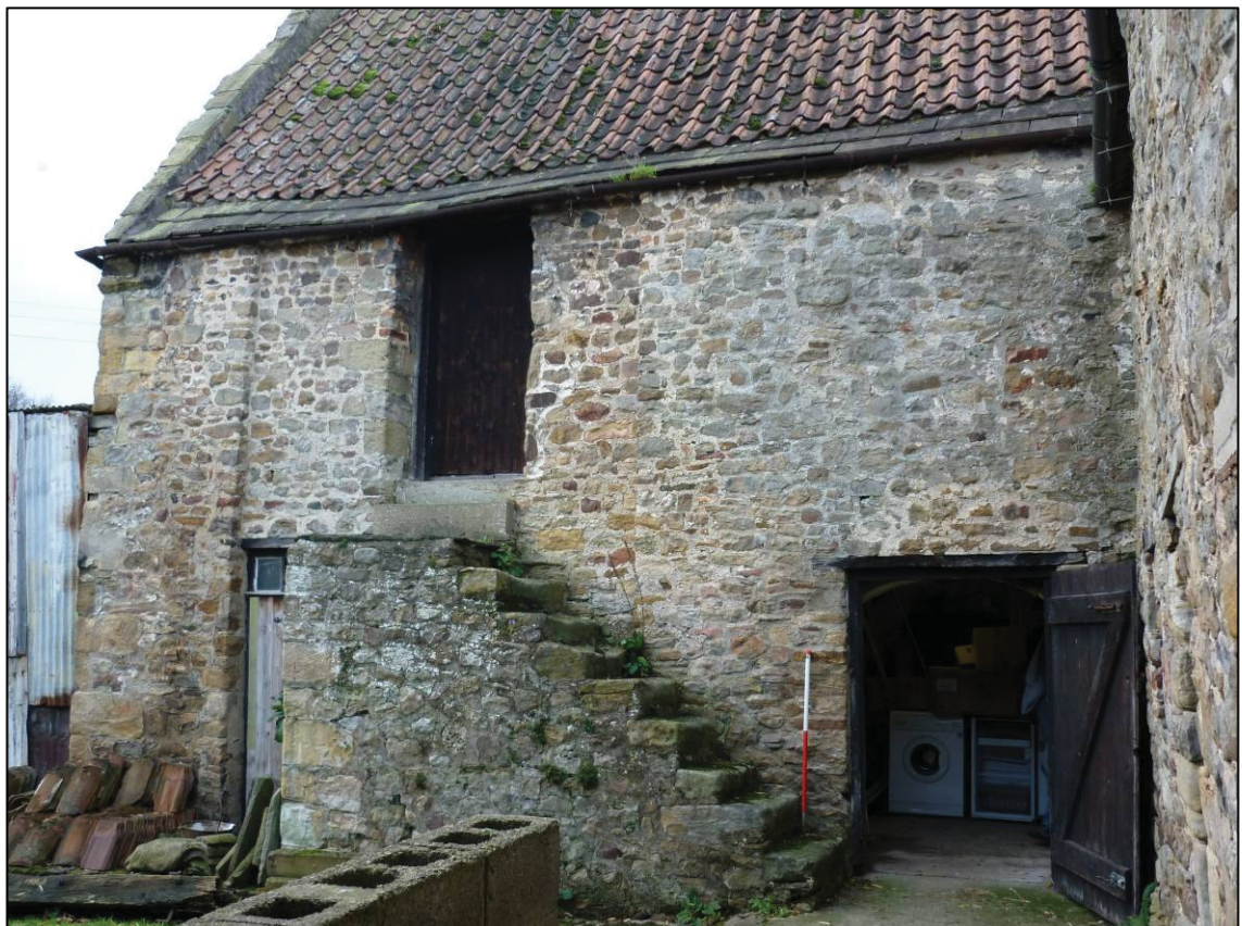
Plate 5: Medieval building, south end of east elevation, looking SW (photo 1/532).
