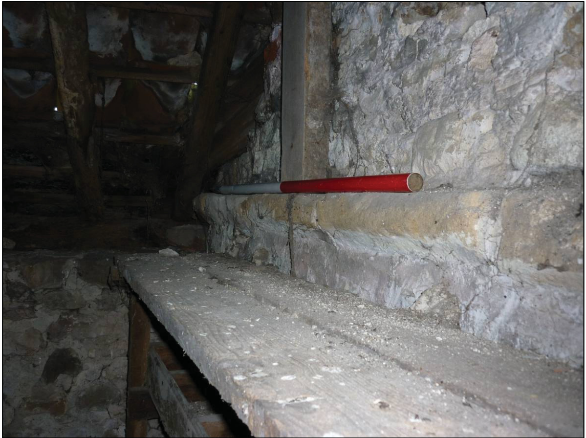
Plate 4: Barn, first floor west cell, showing string course to east elevation of medieval building, looking SW (photo 3/840).
