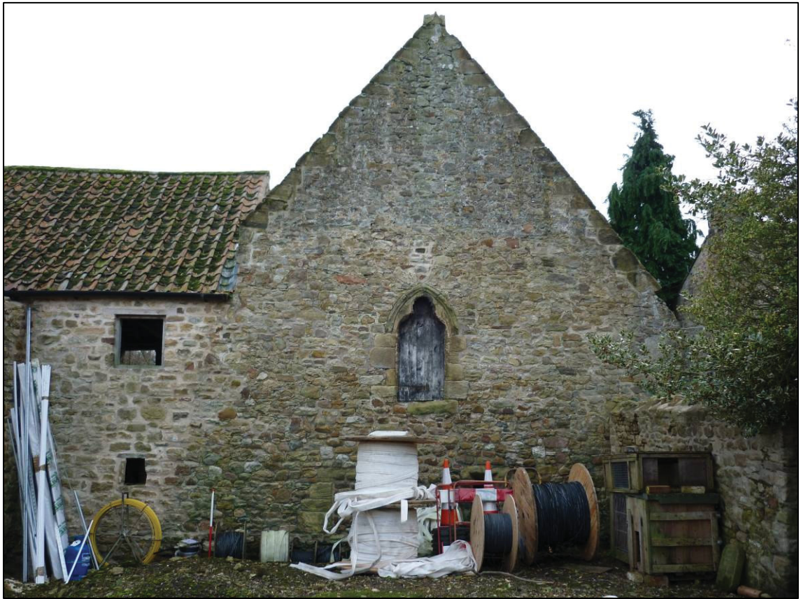
Plate 6: Medieval building, north gable, looking S (photo 1/536).
