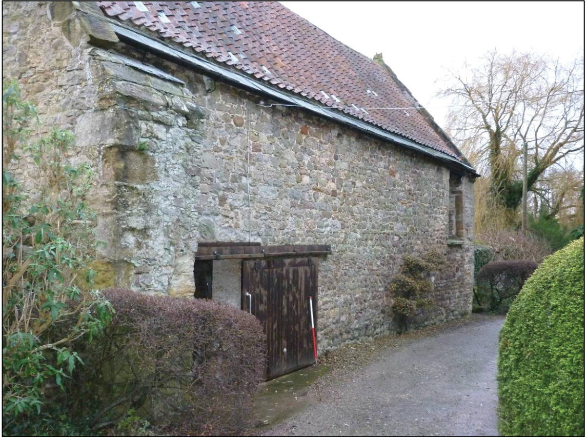
Plate 1: Medieval building, west elevation, looking SE (photo 2/732).
