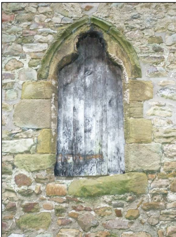
Plate 11: Medieval building, first floor window to north gable, looking S (photo 2/731).
