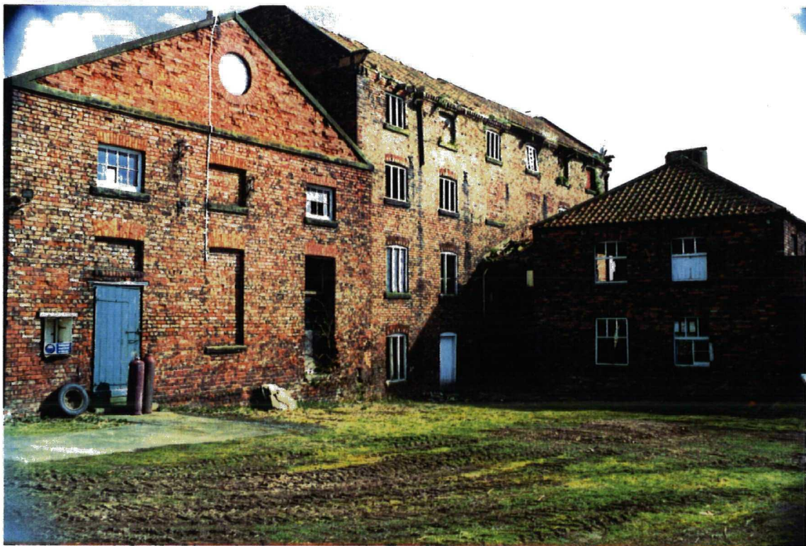
View of King's Mill, facing south-east.
