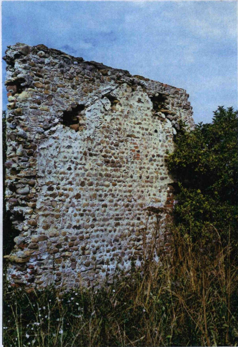
Plate 17. Interior walls of farm building. Facing north-east.
