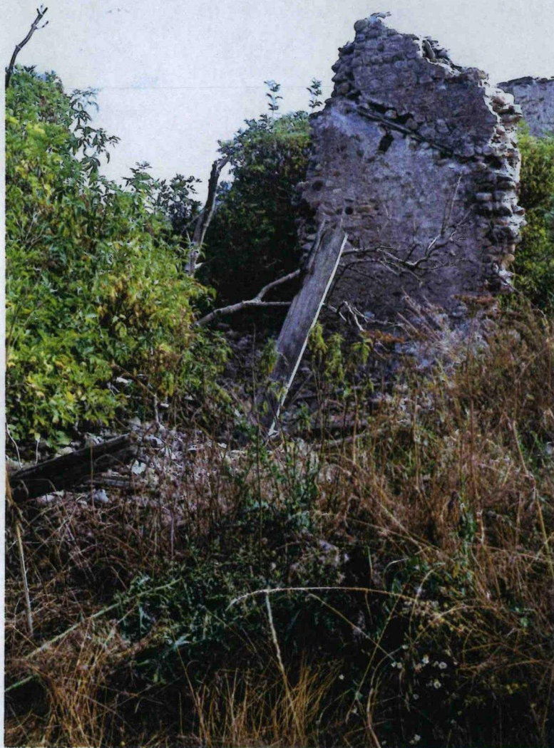
Plate 15. North extent of farm building. Facing south-east.
