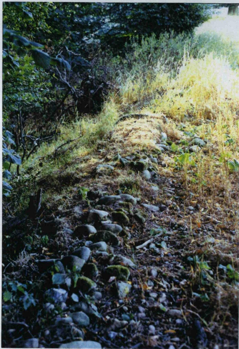
Plate 9. View of wall. Facing west.
