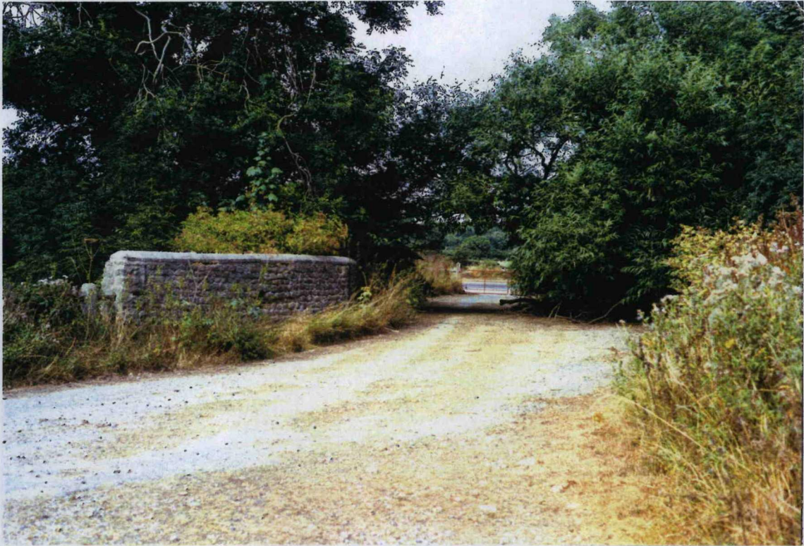
Plate 11. View of Ellerton Bridge. Facing north.
