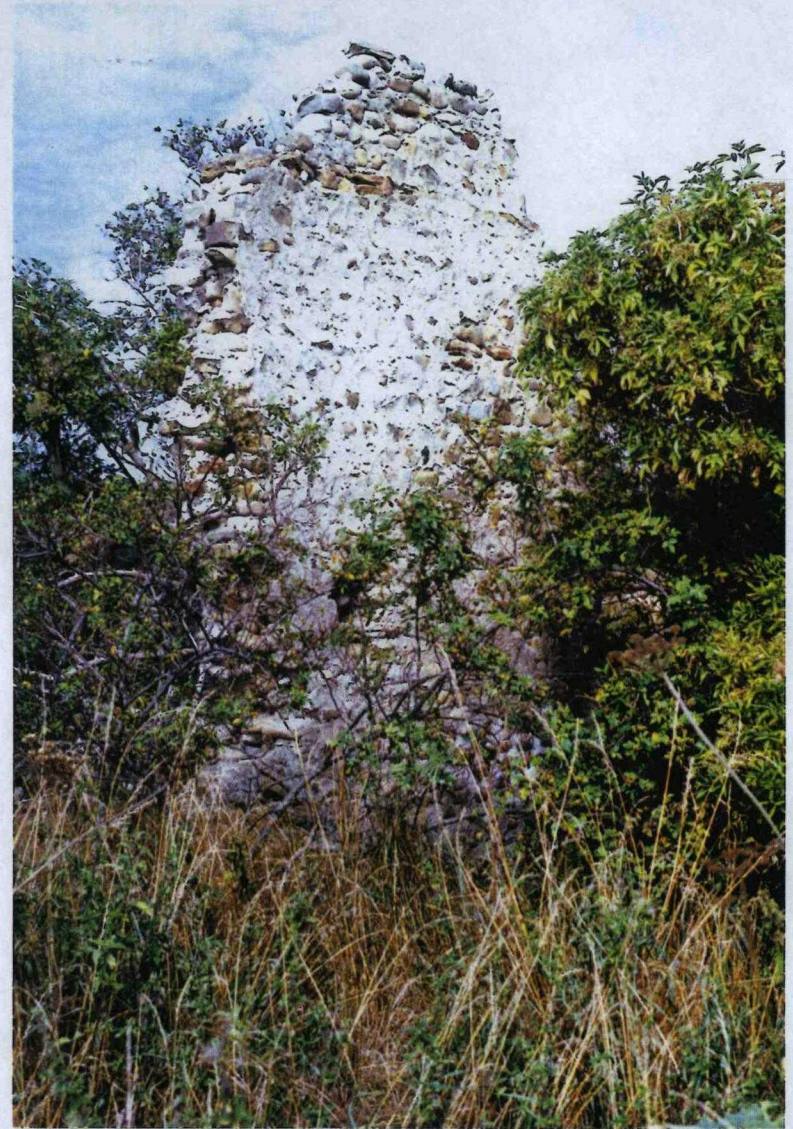
Plate 18. Interior walls of farm building. Facing north-east.
