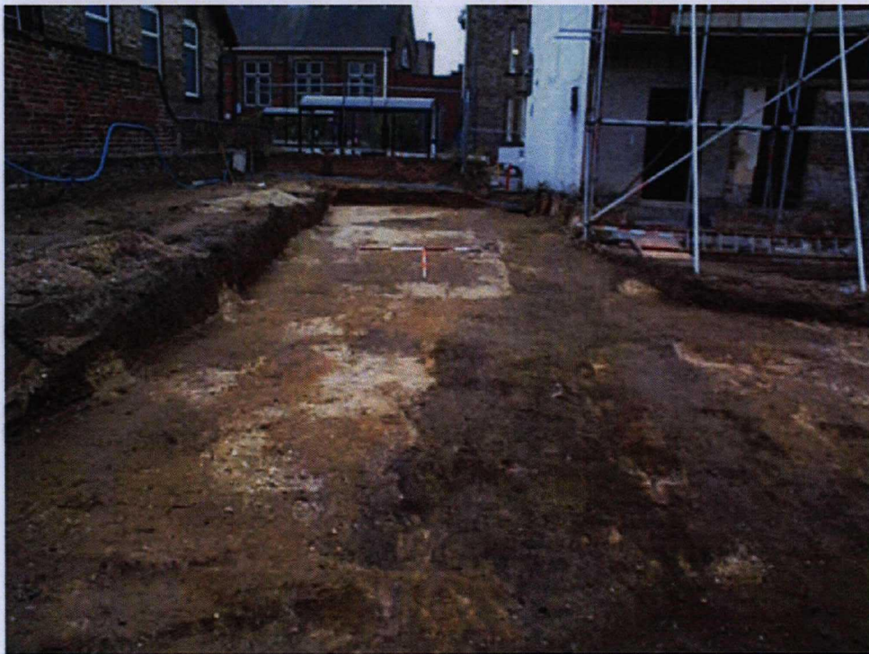
Plate 2. Overall View of Excavation Area. Facing South
