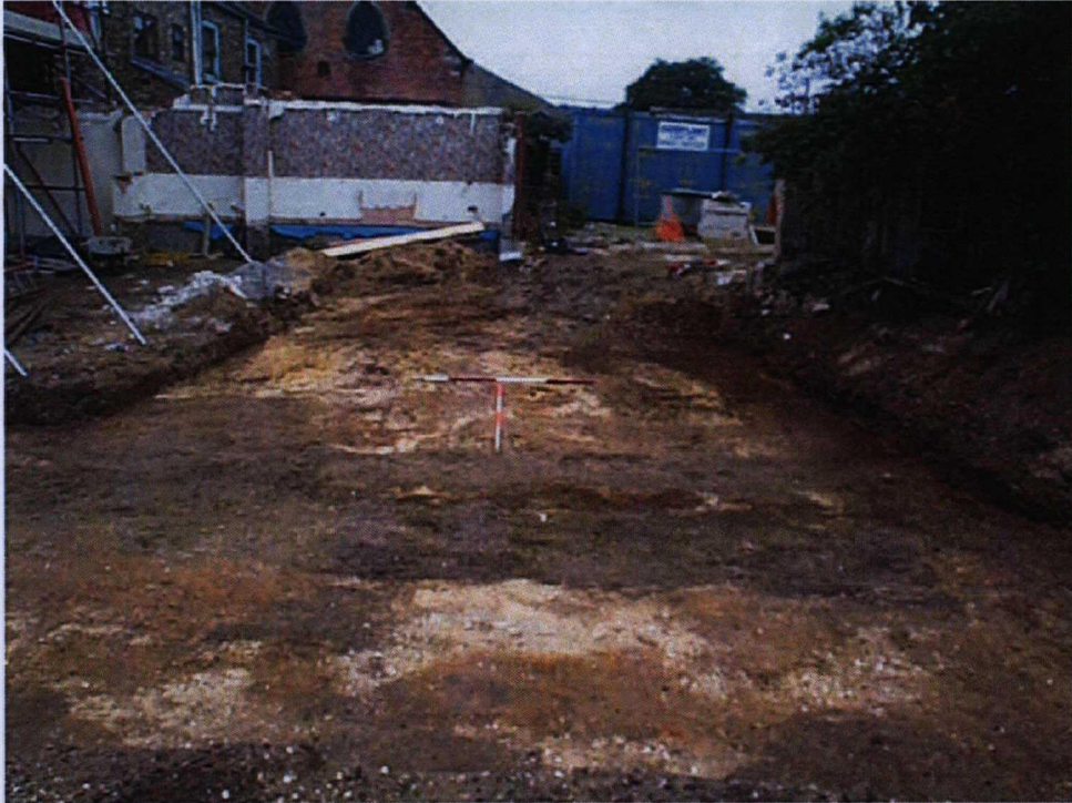
Plate 1. Overall View of Excavation Area. Facing West
