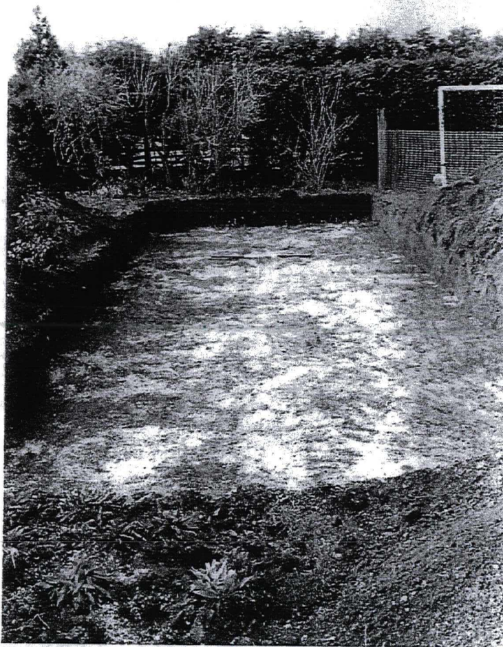
Plate 3. Trench 2 after Cleaning. Facing West
