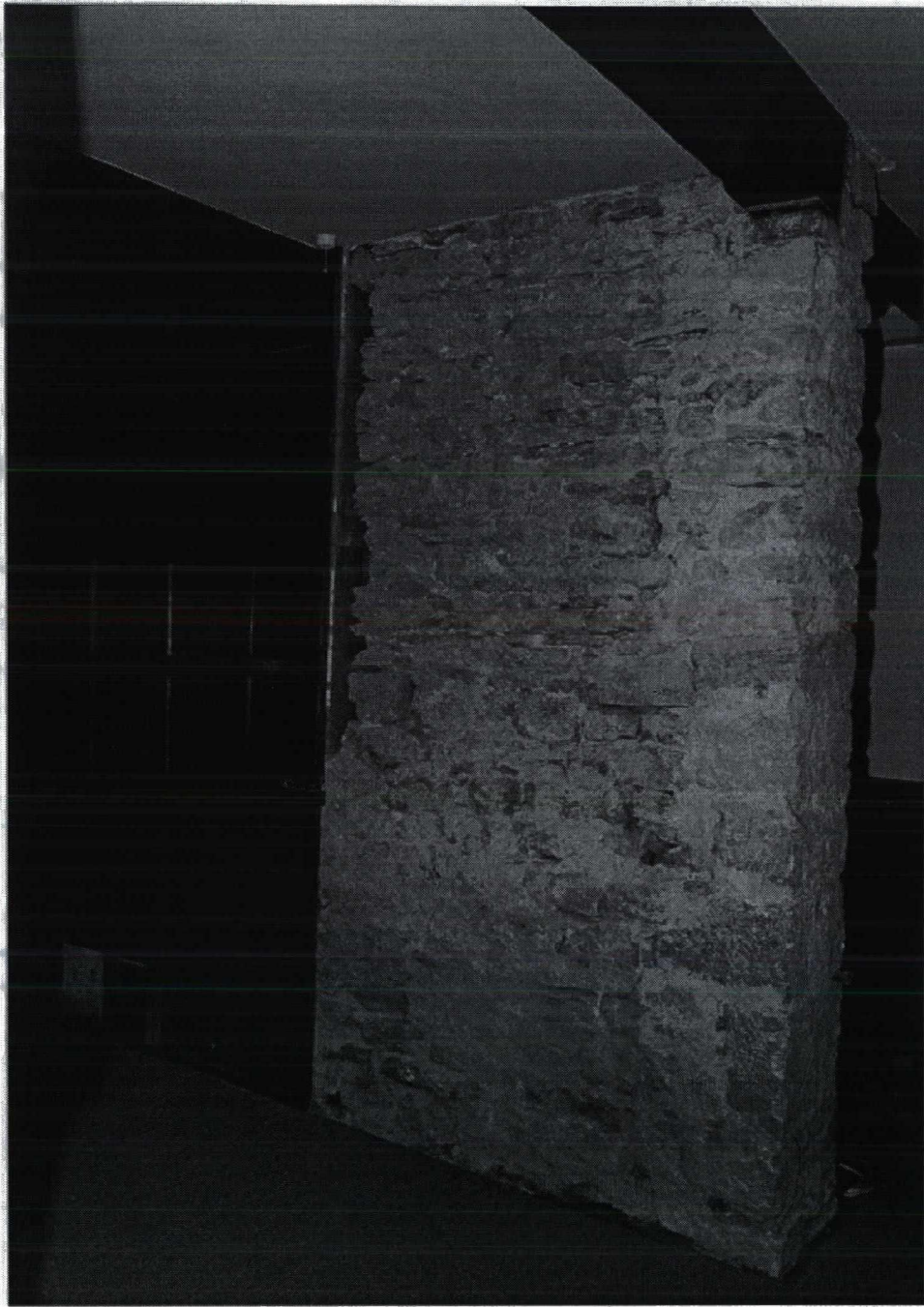
Plate 5 East Face of Passageway Wall Following Removal of Wall Finishes
