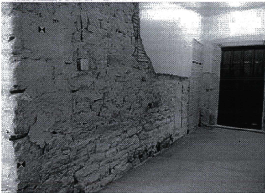
Plate 2 West Face of Passageway Wall – oblique view
