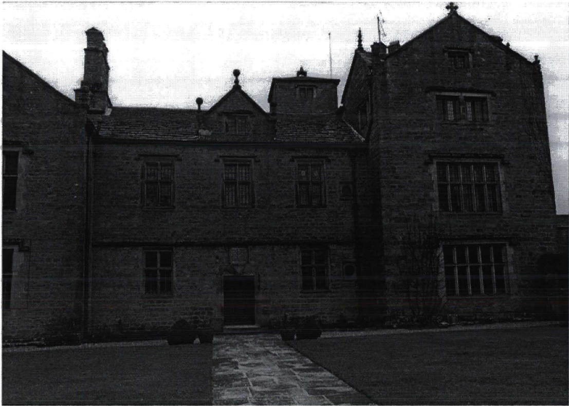
Plate 1 Lawkland Hall Northern Facade
