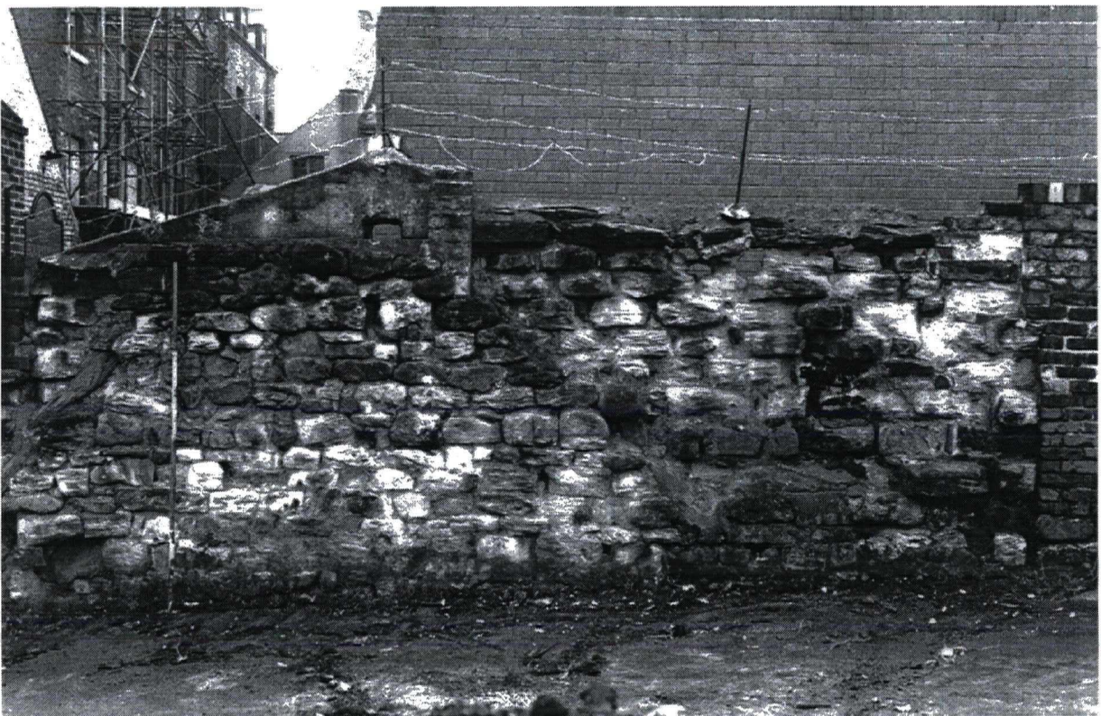
Plate 3: Stone wall forming part of the south boundary of the site
