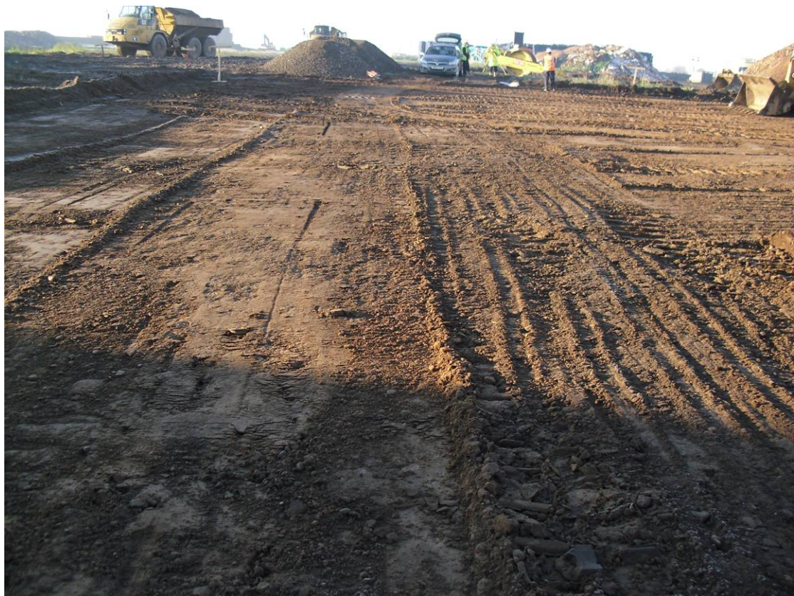
Plate 16: Area 10, initial topsoil stripping
