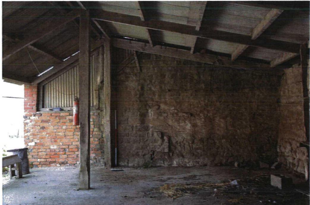
Plate 6 Building 12, internal face of older SE wall with later brick expansion to left. Note old roof line above scale and wall stub to right of this. Looking SE
