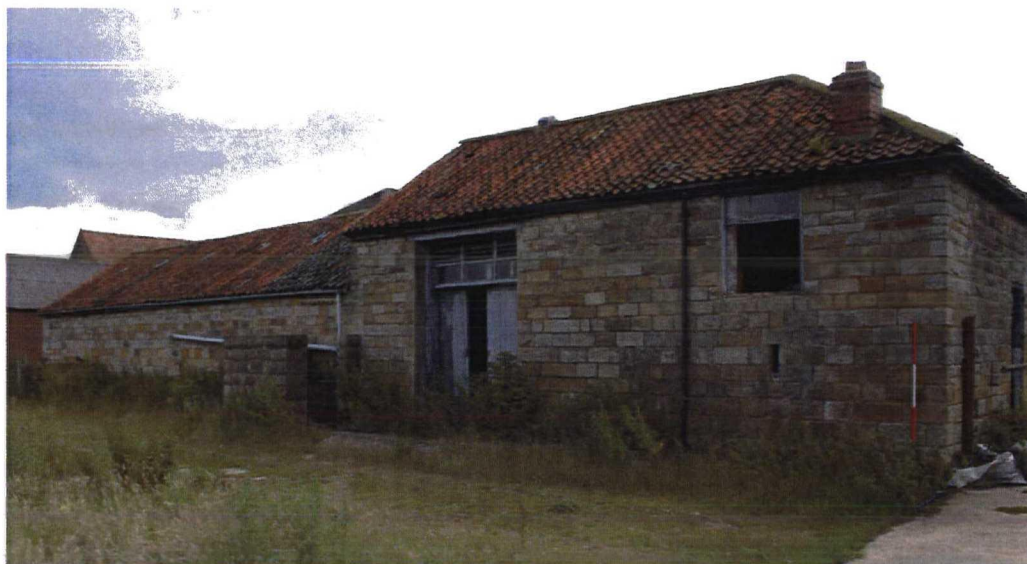
Plate 3 Building 10 with taller N end. Looking SSW
