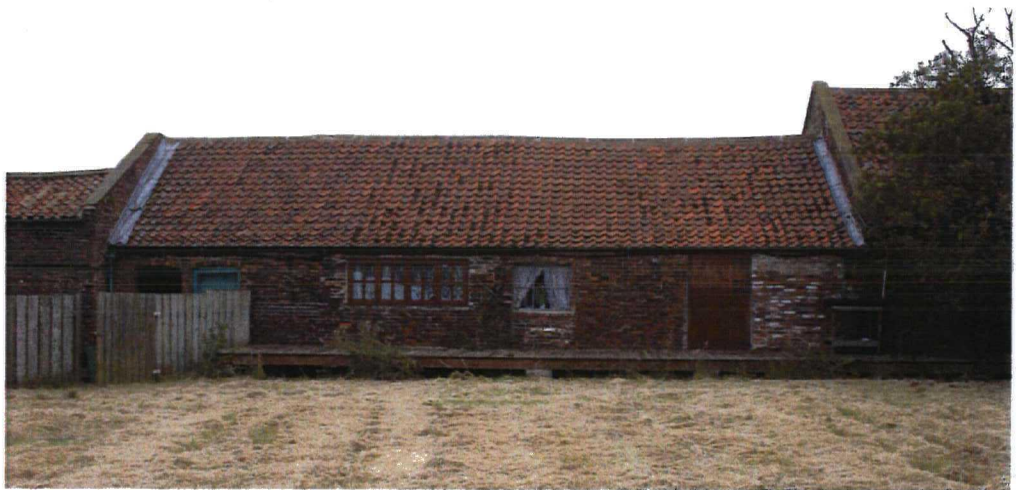
Plate 16 Building 20, E elevation. This side of the building built (or re-built) in brick. Building 19 to right, Building 21(C) to left in area of green door. Looking W
