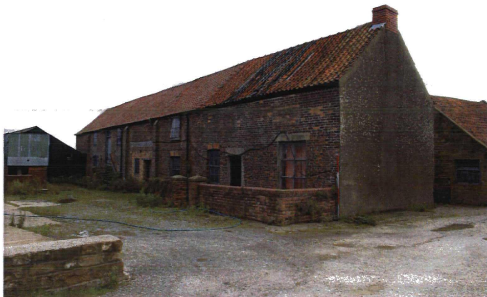
Plate 13 Building 15, N elevation – dwelling (A) to right and barn (B) to left. Note large blocked opening of barn door. Looking E
