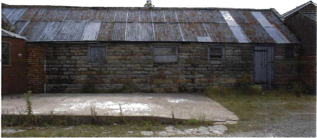
Plate 7 Building 13, E elevation. Looking WSW
