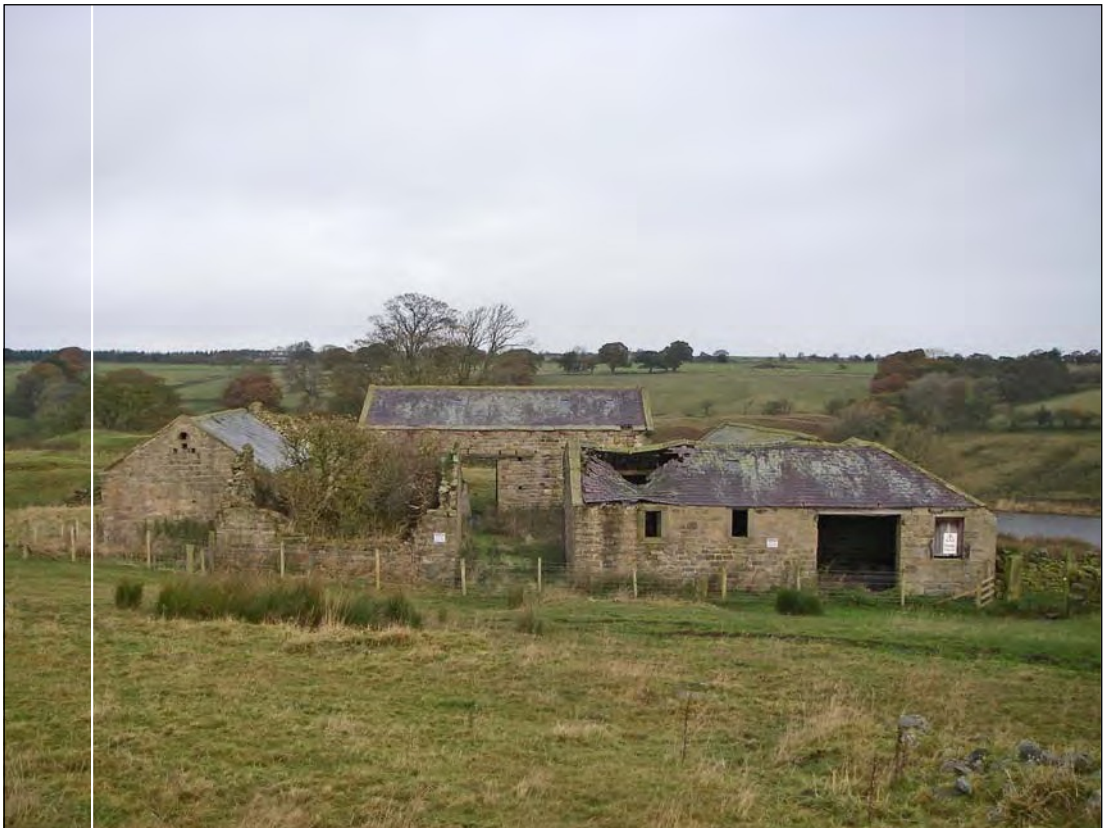
Plate 8. The southern side of the farm building range, looking north
