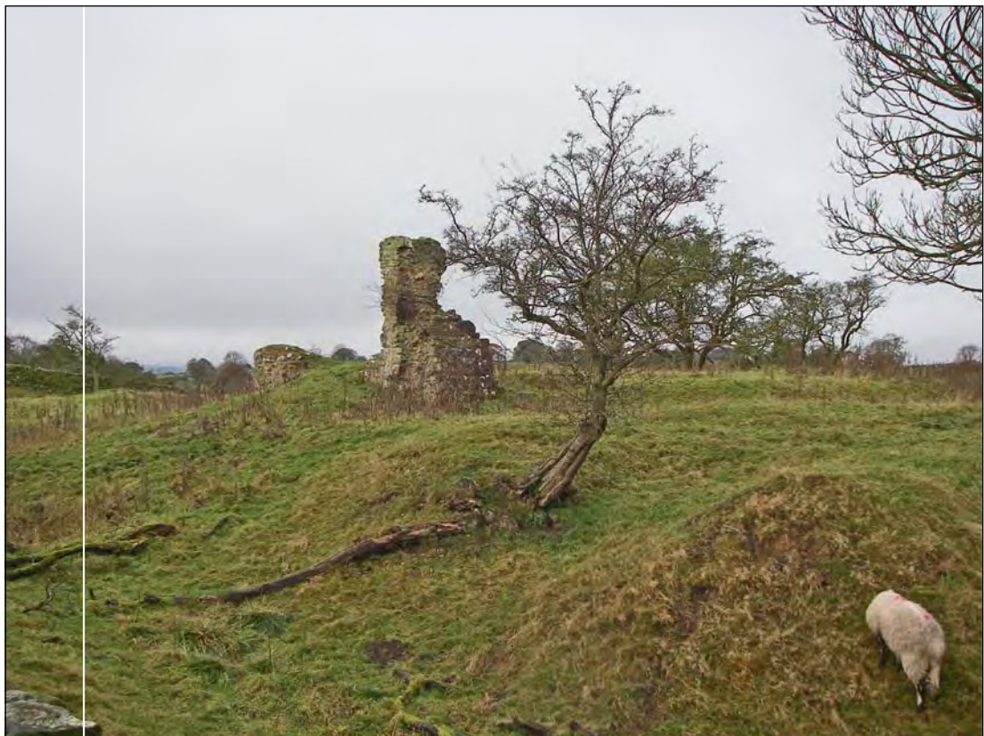
Plate 4. The south-western corner of the moat of 'John of Gaunt's Castle' with the remains of the gatehouse situated on its southern side, looking west
