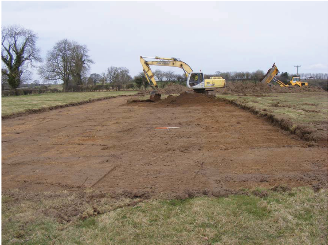
Plate 1. Stripping of Western Side of Site. Facing North-East
