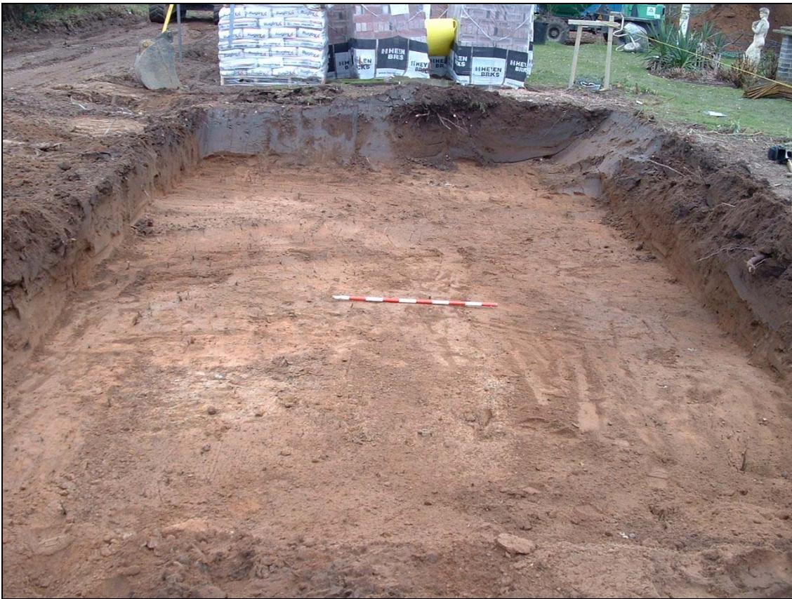
Plate 1. Typical view of southern end of Trench 1.
