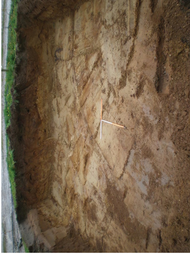
Plate 3. Wind Turbine Base at Formation Level. Facing West.
