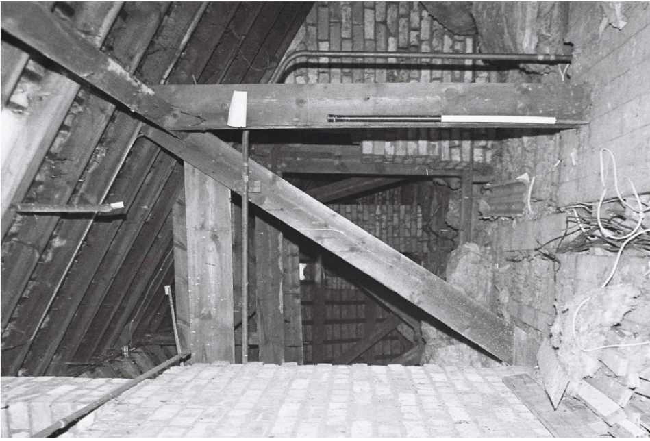
Plate 47. Oak Mount: Interior Attic. Facing West.
