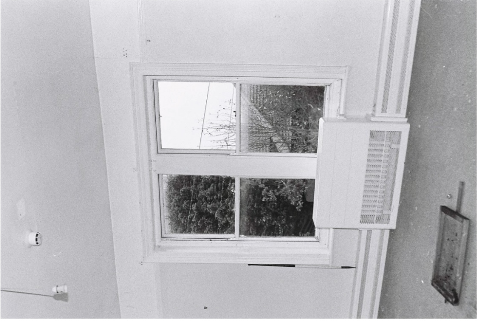
Plate 34. Oak Mount: Interior First Floor. Facing South.
