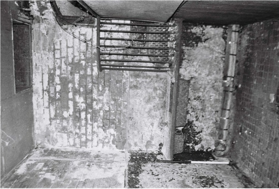
Plate 79. Stables: Interior Ground Floor. Facing East.
