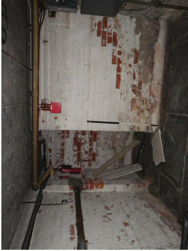
Plate 49. Oak Mount: Interior Cellar. Facing South.
