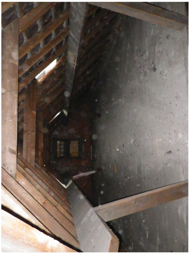
Plate 84. Stables: Interior Hayloft. Facing North.
