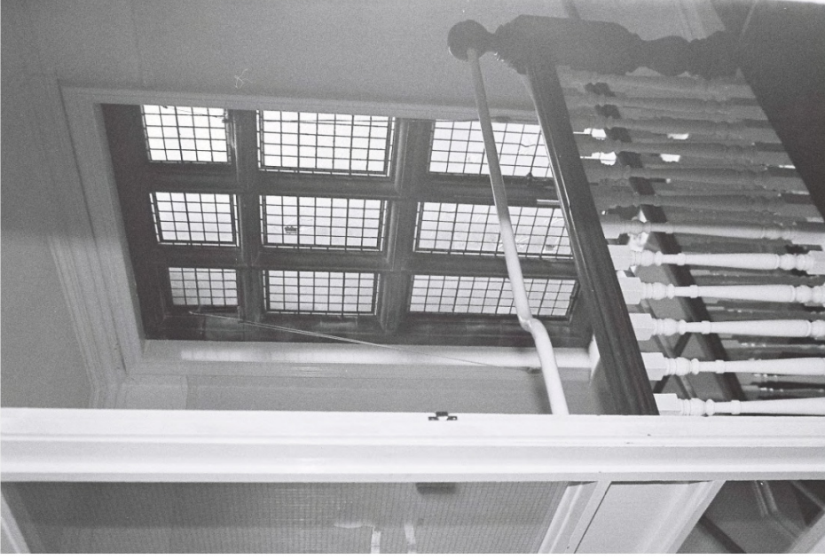
Plate 25. Oak Mount: Interior First Floor. Facing North-west.
