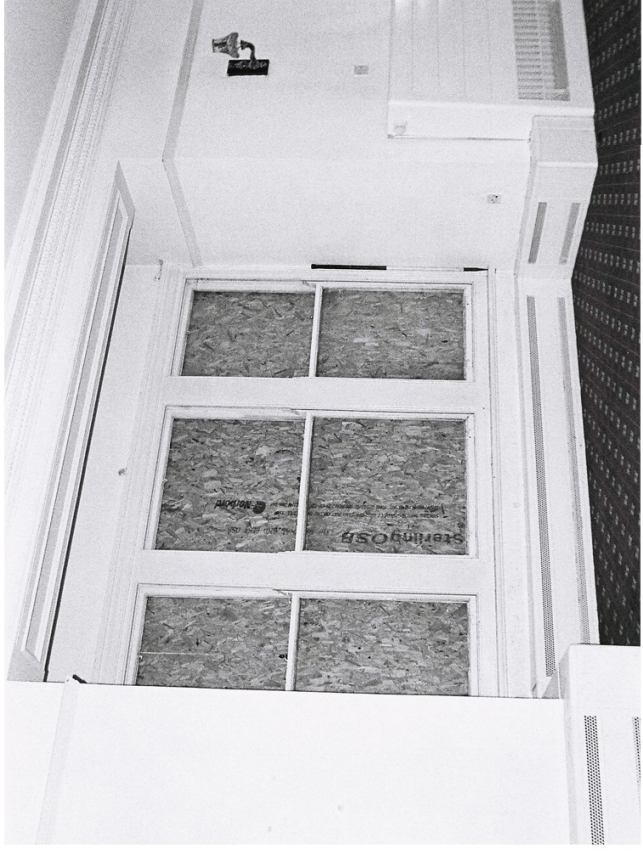
Plate 14. Oak Mount: Interior Ground Floor. Facing West.
