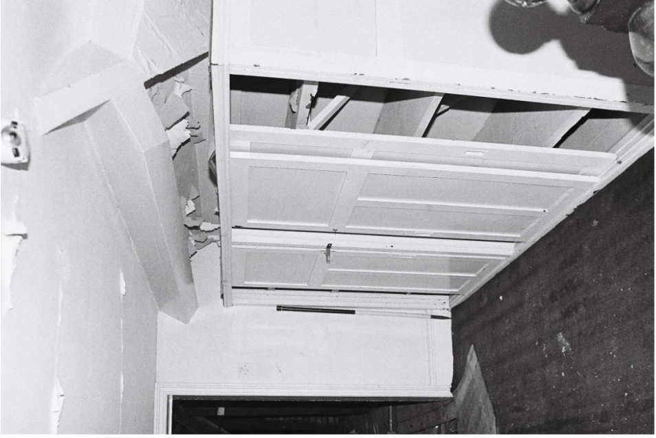
Plate 46. Oak Mount: Interior Attic. Facing West.
