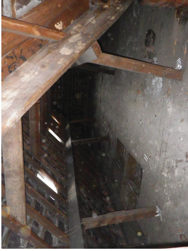
Plate 86. Stables: Interior Hayloft. Facing South.
