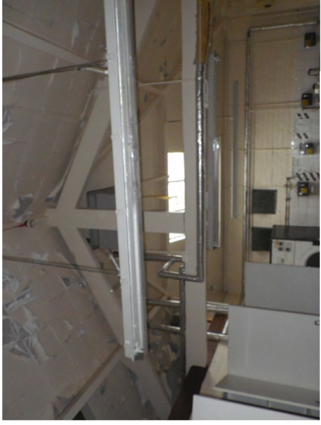
Plate 56. Outbuilding: Interior. Facing South.
