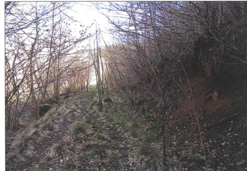
Plate 12. View of footpath and damage to earthen banks
