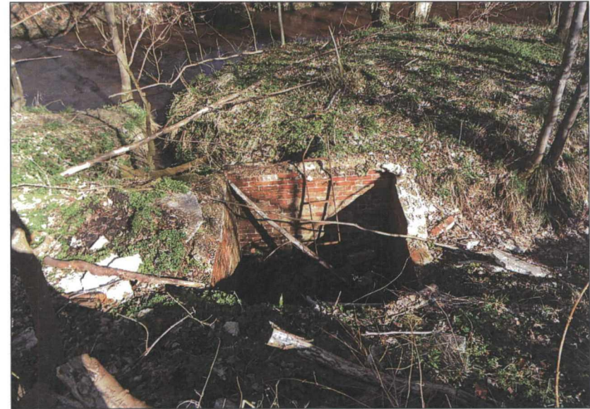
Plate 10. View of modern brick structure identified during walkover survey
