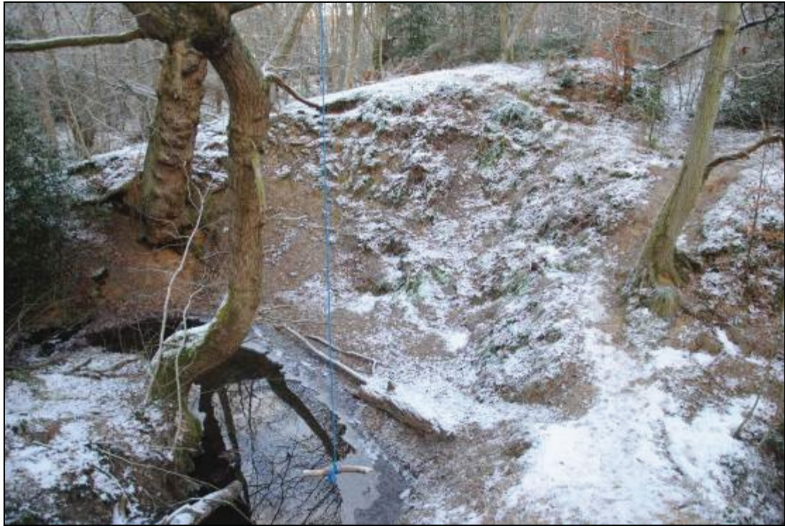
Figure 20 The breach in the west dam, looking north-east
