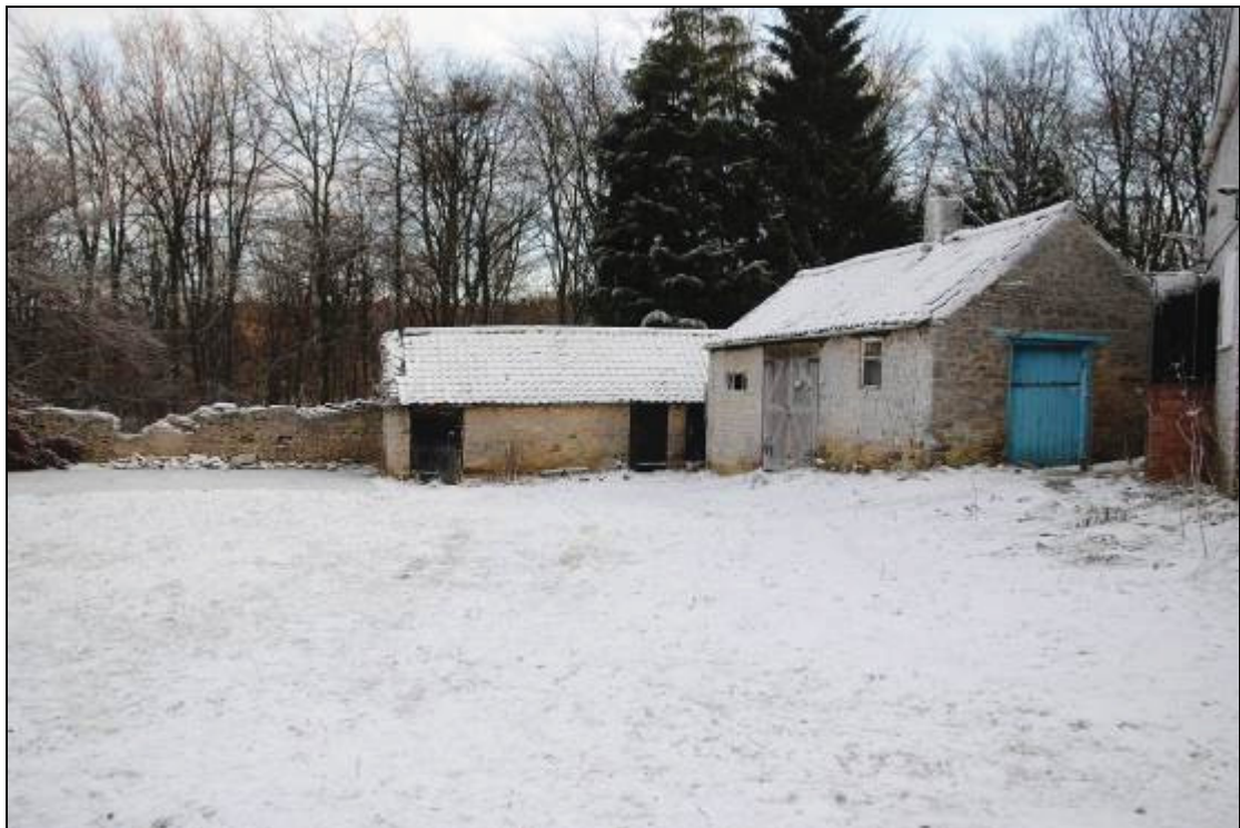
Figure 11 Windy Gate Farm; the south and east outbuildings
