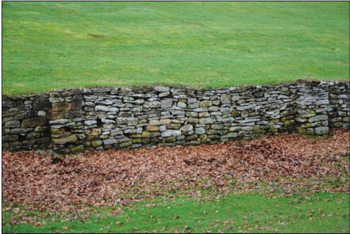
Figure 8 The ha-ha wall below the terraces
