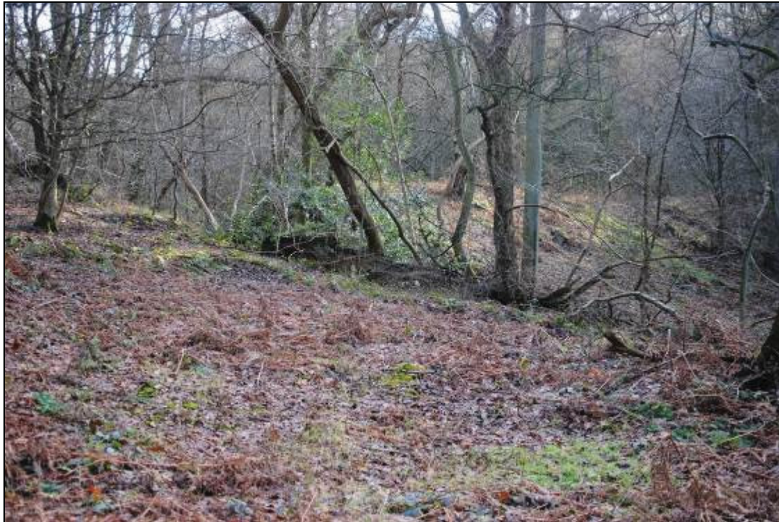
Figure 24 The north face of the east dam and the breach, looking south-east
