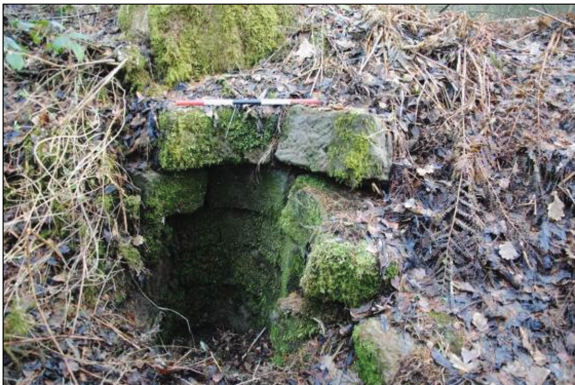
Figure 25 The stone-lined shaft in the east dam; 0.5m scale
