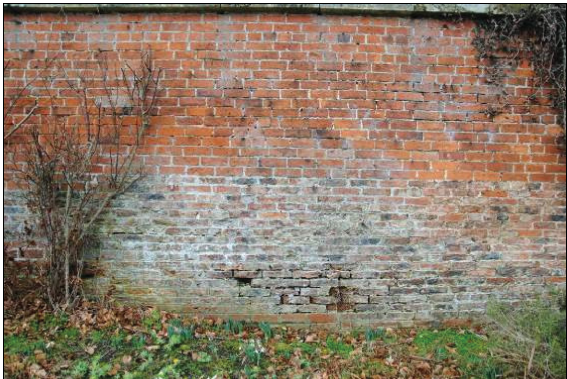
Figure 7 Detail of the retaining wall on the lower terrace
