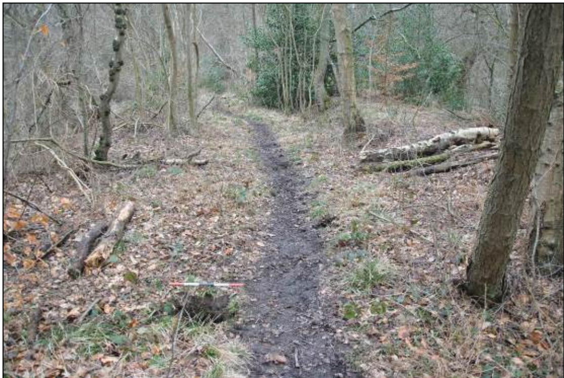
Figure 21 Looking west along the path on the west dam. The small hole in the left foreground is the stone shaft, and the bank to the right the crest of the dam wall
