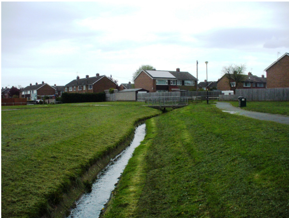
Plate 3: general view of Turker Beck in Bullamoor Park looking northeast towards Turker Close, showing the artificially graded banks
