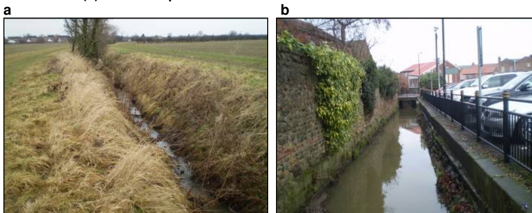
Figure 2.1: Examples of channel modification, (a) re-sectioning and straightening – Turker Beck (b) hard bank protection – Sun Beck.
