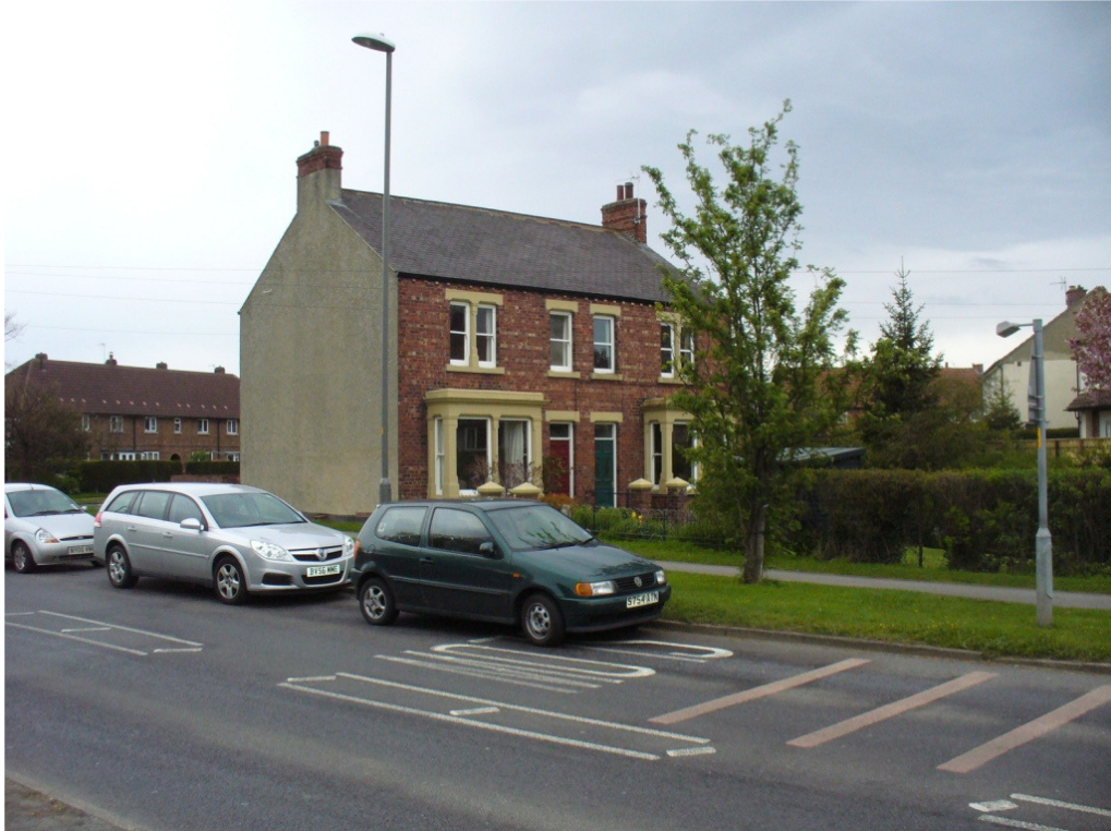
Plate 5: the Victorian houses to the south of Bullamoor Road (Asset 21)
