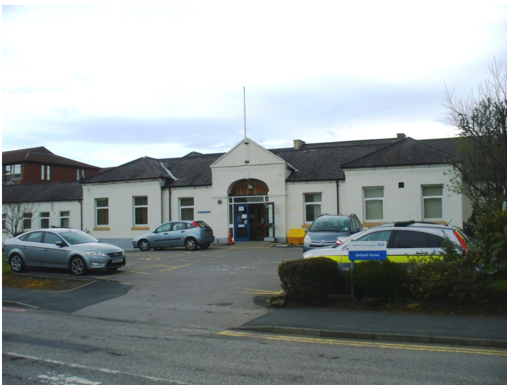
Plate 4: the Northallerton Union Workhouse (Asset 17)
