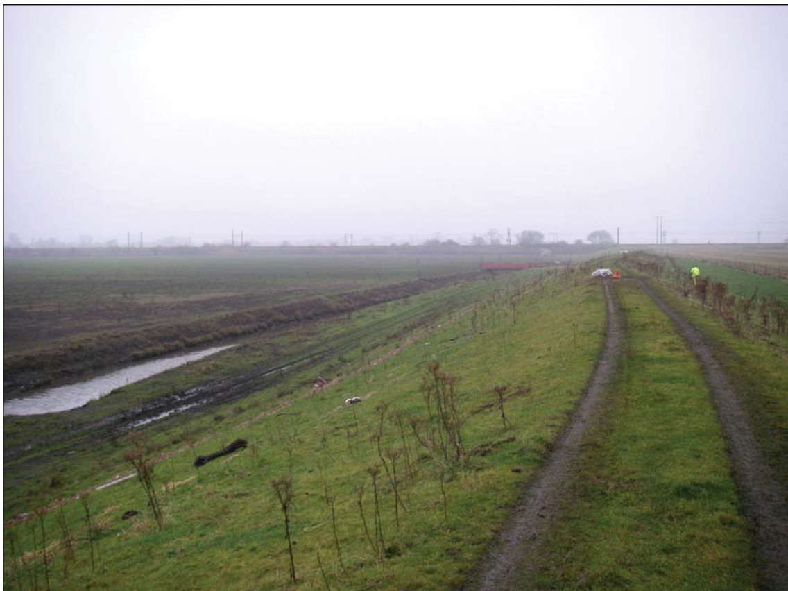
Plate 2. View along Sea Bank and Ings and Tetherings Drain, facing east
