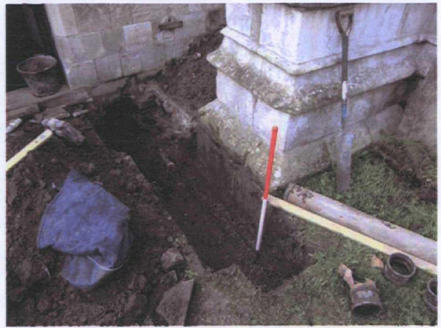
Plate 5 Foul drainage pipe looking SW
