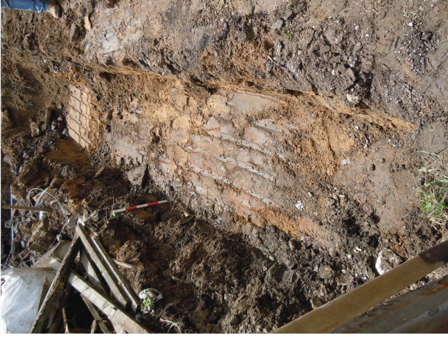
Plate 4. Foundation of Boundary Wall. Facing South.
