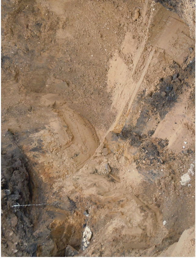
Plate 2. Soakaway. Facing North-west.
