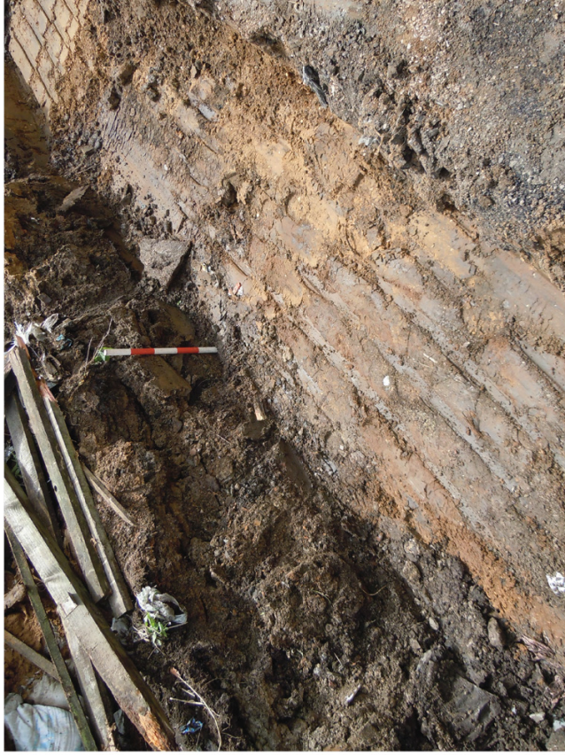
Plate 3. Foundation of Boundary Wall. Facing South-east.
