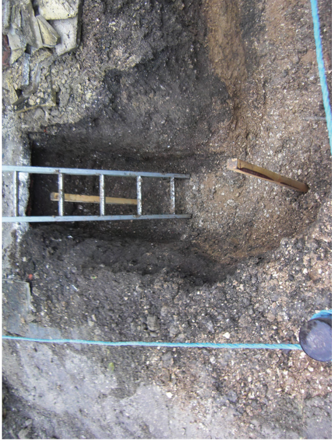
Plate 1. View of Foundation Trench. Facing South.
