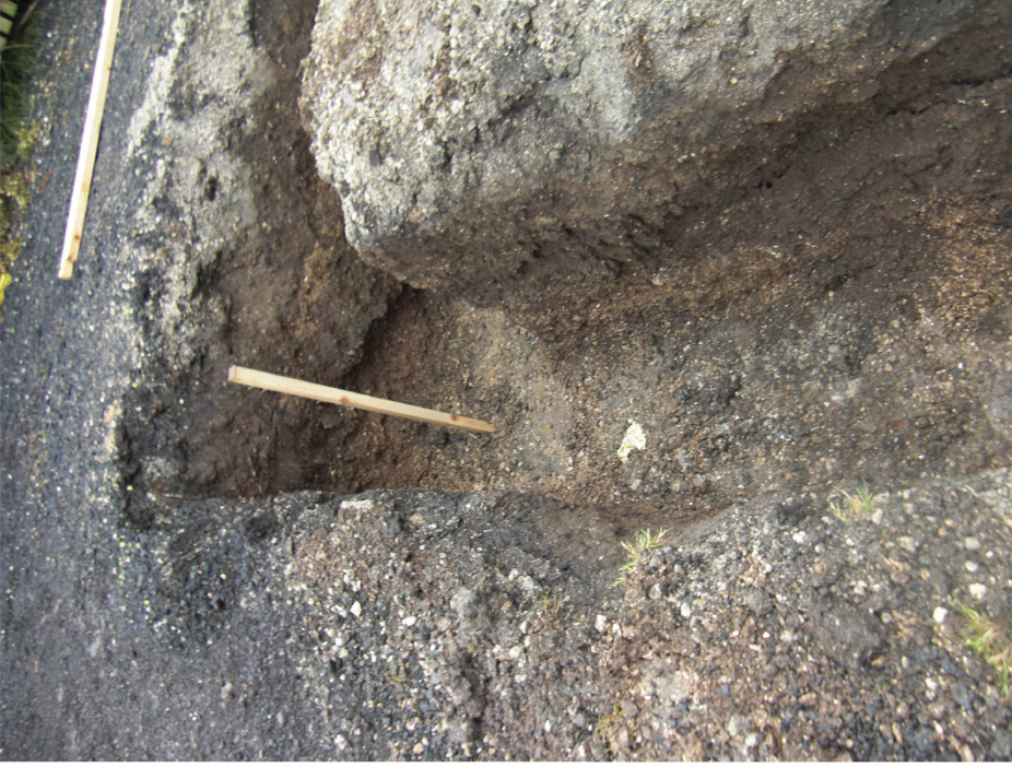
Plate 3. View of Foundation Trench. Facing West.
