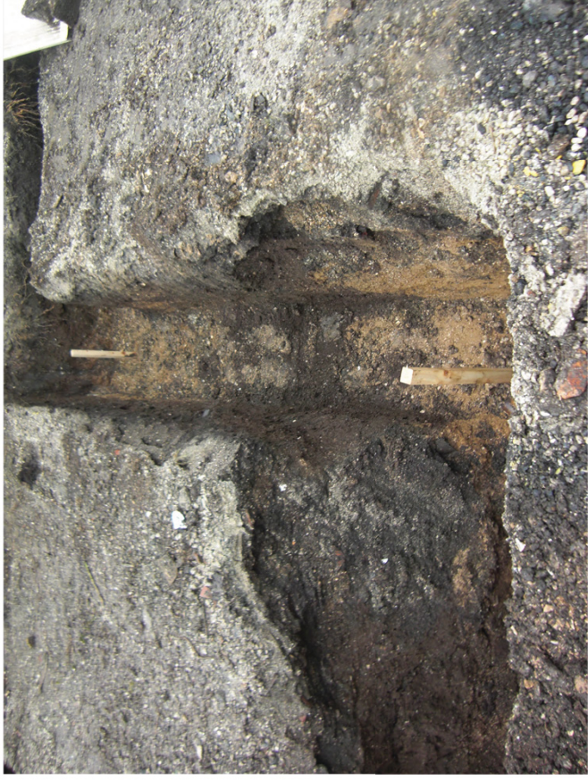
Plate 2. View of Foundation Trench. Facing South.
