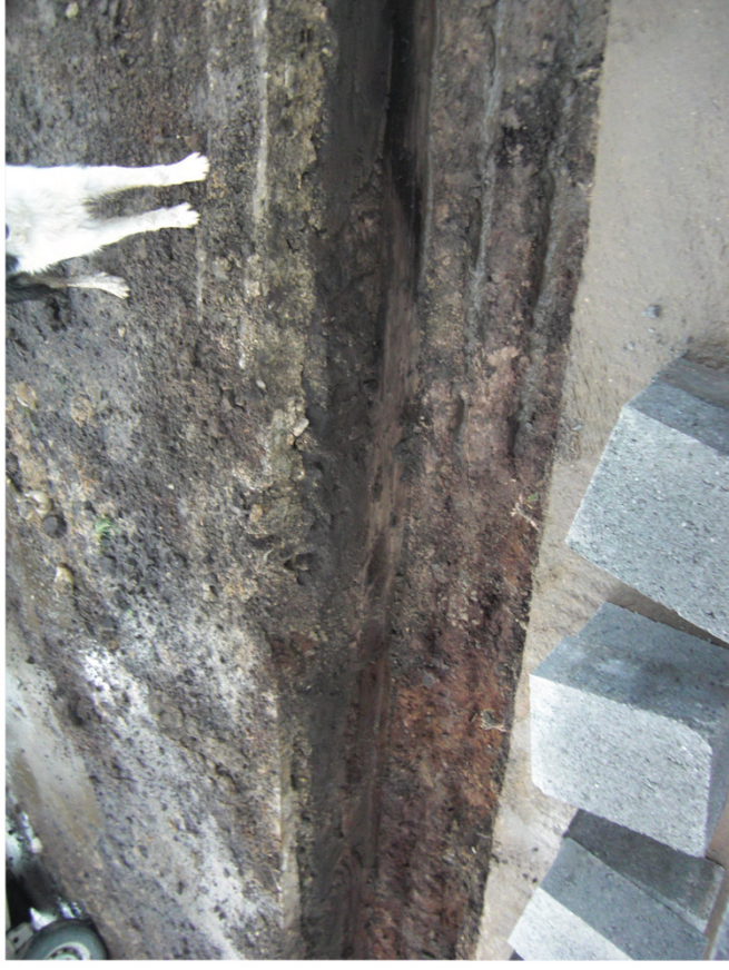
Plate 4. View of Foundation Trench. Facing North-West,
