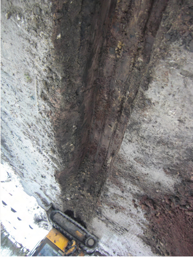
Plate 2. View of Foundation Trench. Facing South-west.
