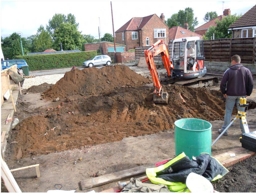
Plate 1. General View of Site Pre-excitation. Facing North-east.
