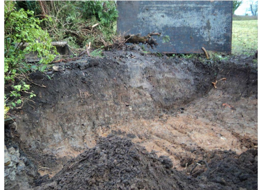
Plate 4. Section through Stripped Area. Facing North-east.
