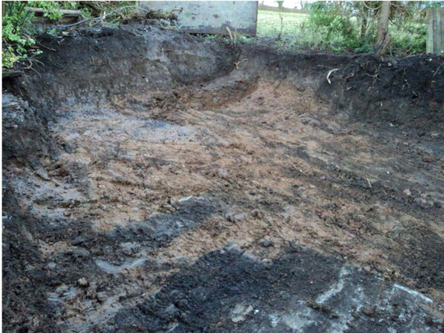
Plate 3. View of Stripped Area for Extension. Facing North.
