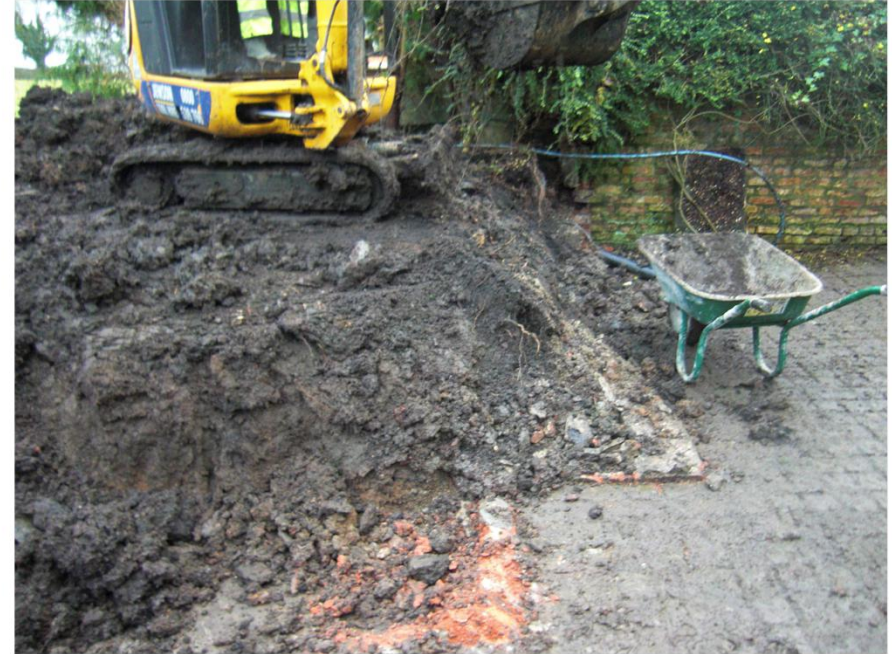
Plate 2. Area during ground reduction. Facing North.
