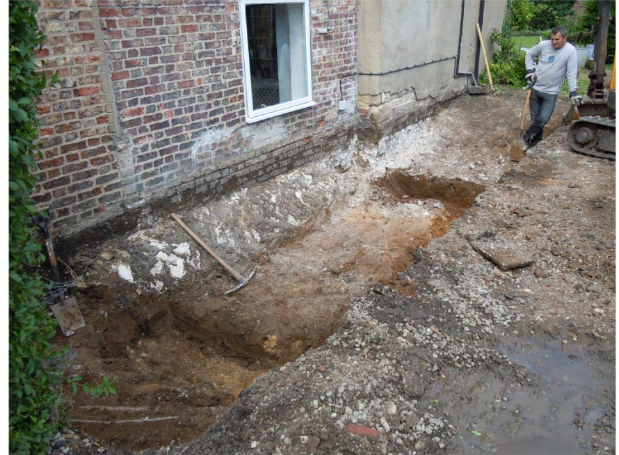
Plate 4. Completed site. Facing North-east.
