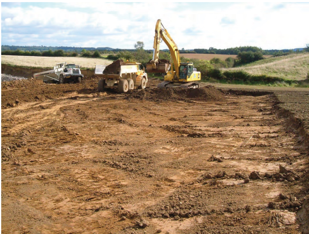
Plate 2. View of Topsoil Strip. Facing South East
