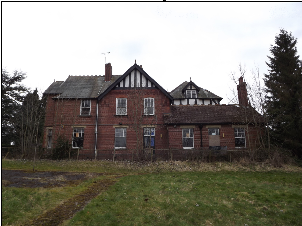
Plate 2. View of the rear (eastern) elevation of Red House.
