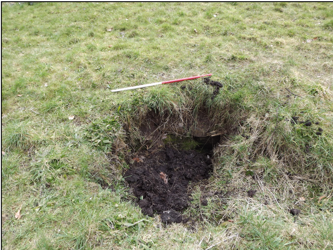
Plate 5. Exposure of buried structure on the northern edge of the platform, scale 1m, looking south.
