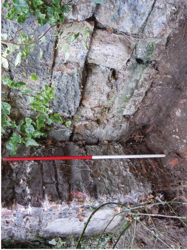
Plate 3. Over-lapping Stone and Brick Walls. Facing North West.
