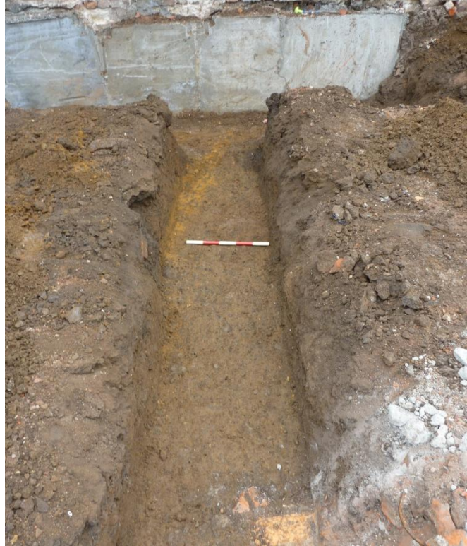
Plate 6 Ditch 3316 / 3548 showing in base of new foundation trench. Yellow natural showing top left of scale. Looks east. 0.10m scale units.
