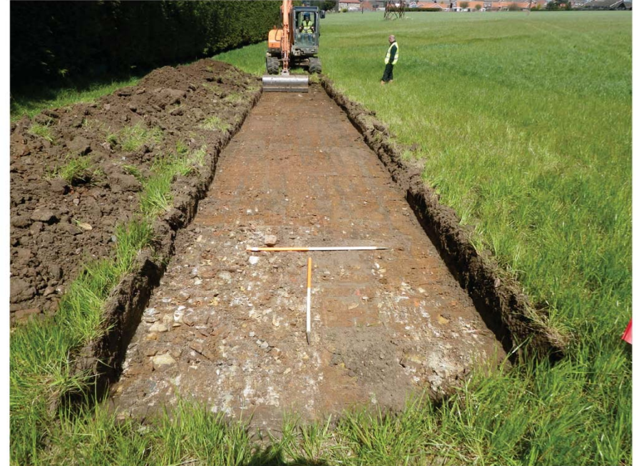
Plate 18. Evaluation Trench 11. Facing North.
