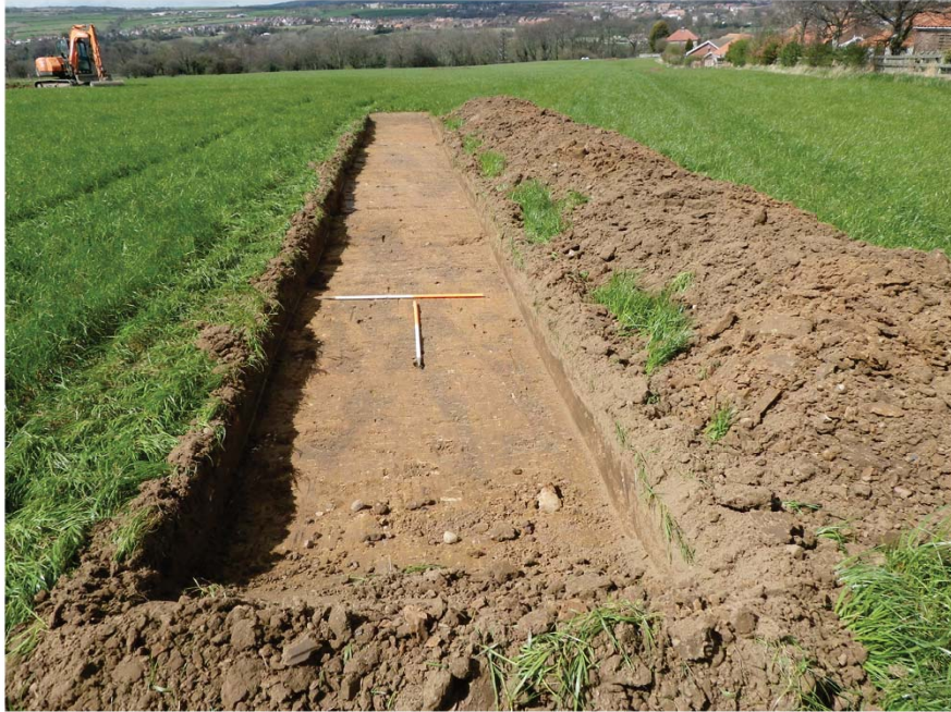
Plate 11. Evaluation Trench 4. Facing West.
