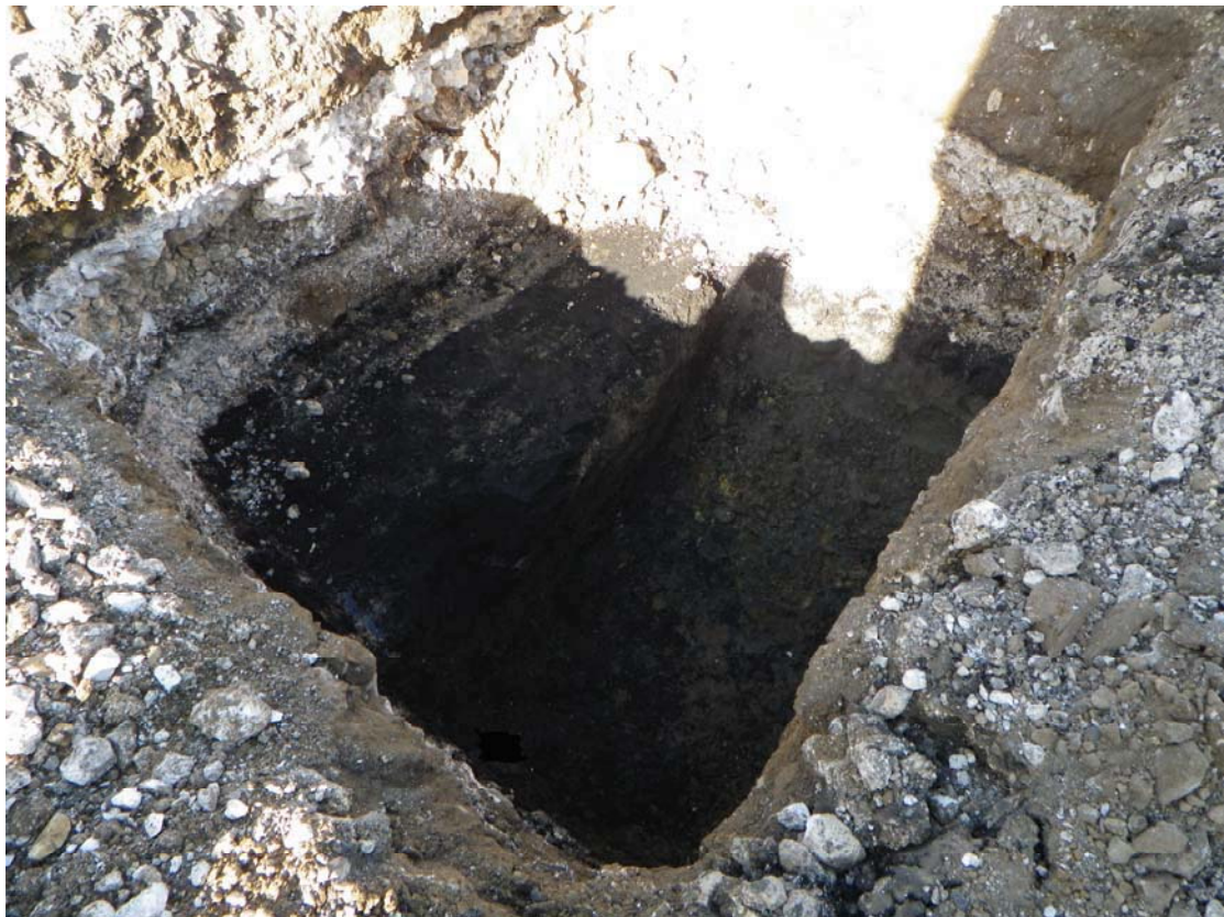
Plate 4 Trial Pit 3 under excavation, looking east
