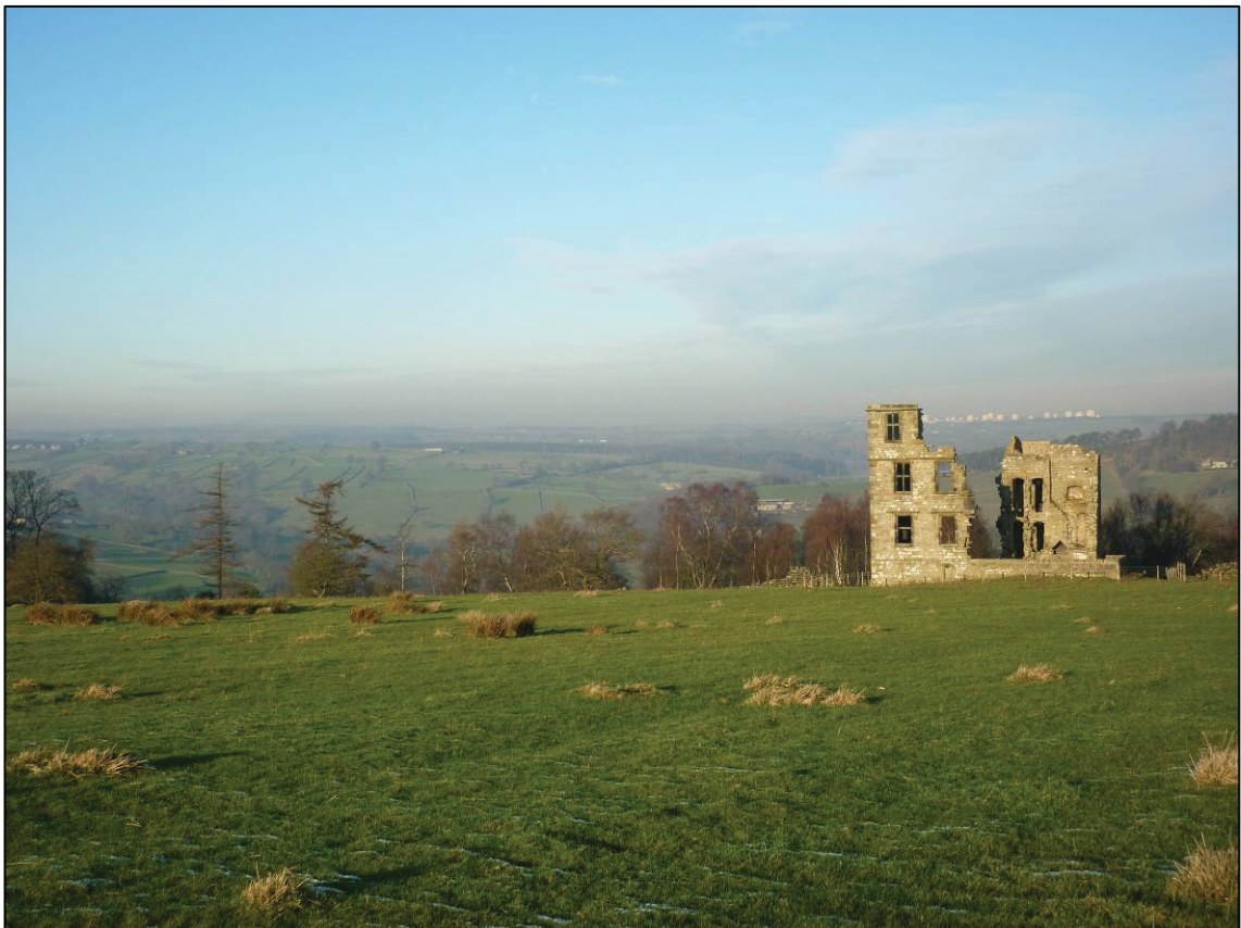
Plate 2: Dobpark Lodge, looking NE (photo 1/348).
