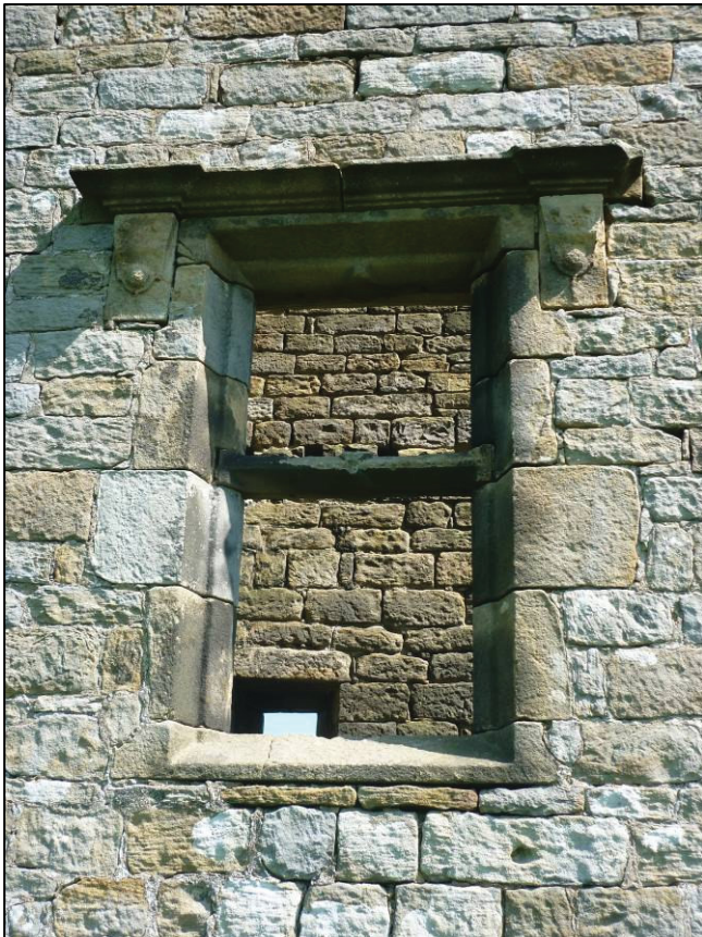
Plate 12: Window W14 in elevation 11 (photo 3/205).
