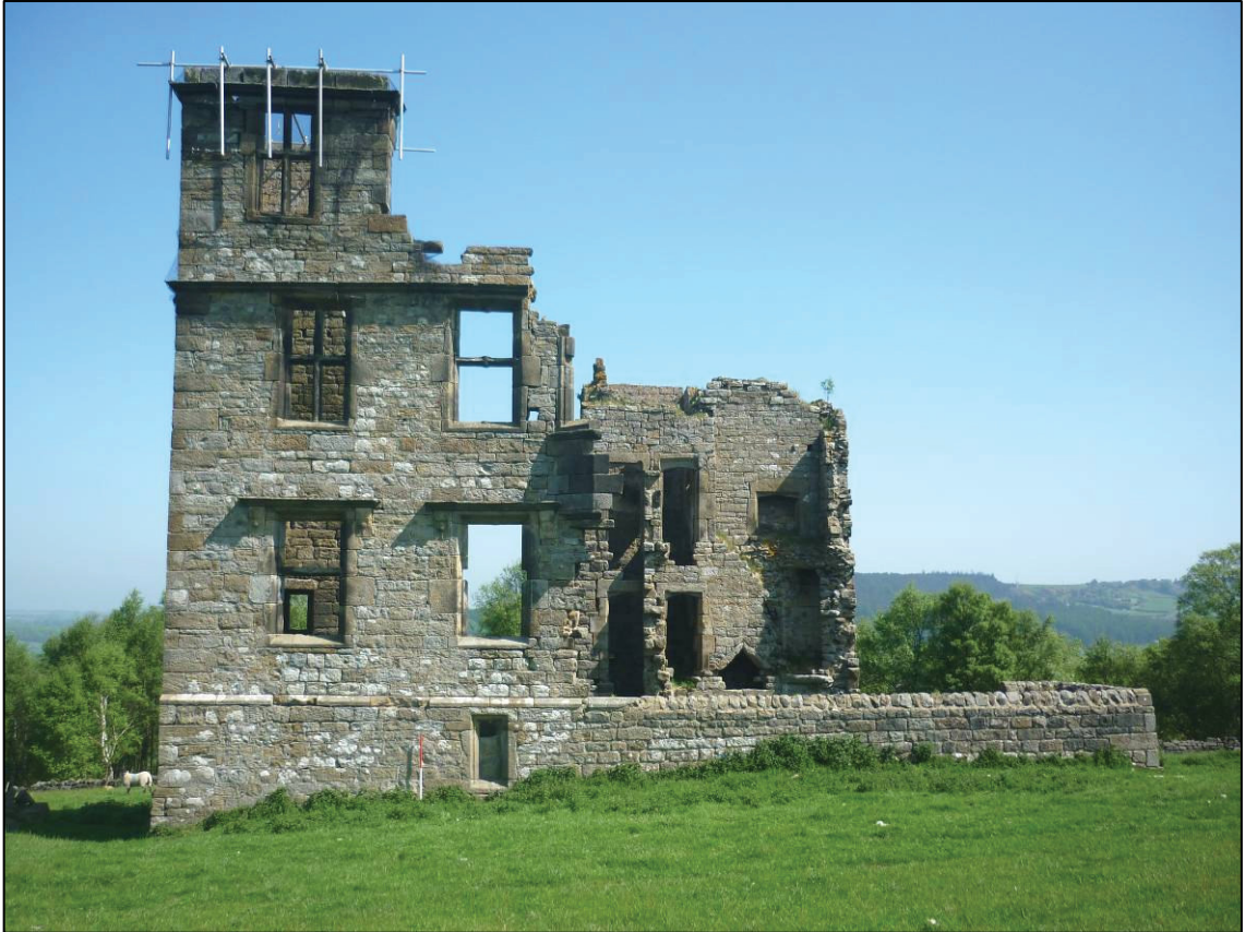
Plate 1: Dobpark Lodge, looking NE (photo 3/203).
