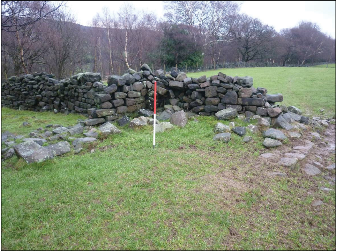
Plate 5: Structure in wall to east of lodge, looking SE (photo 2/498).
