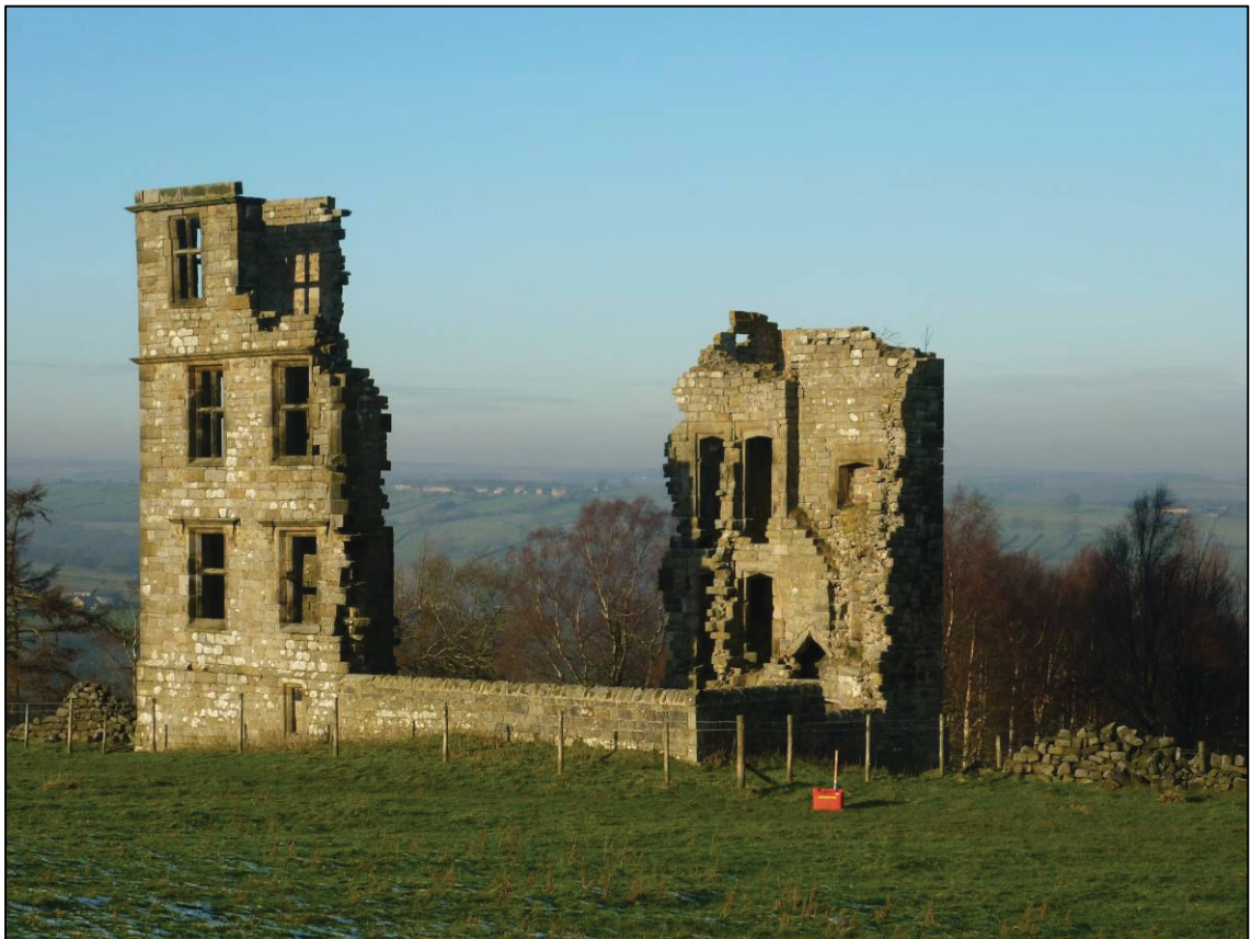
Plate 23: General view to Dobpark Lodge, looking N (photo 1/324).
