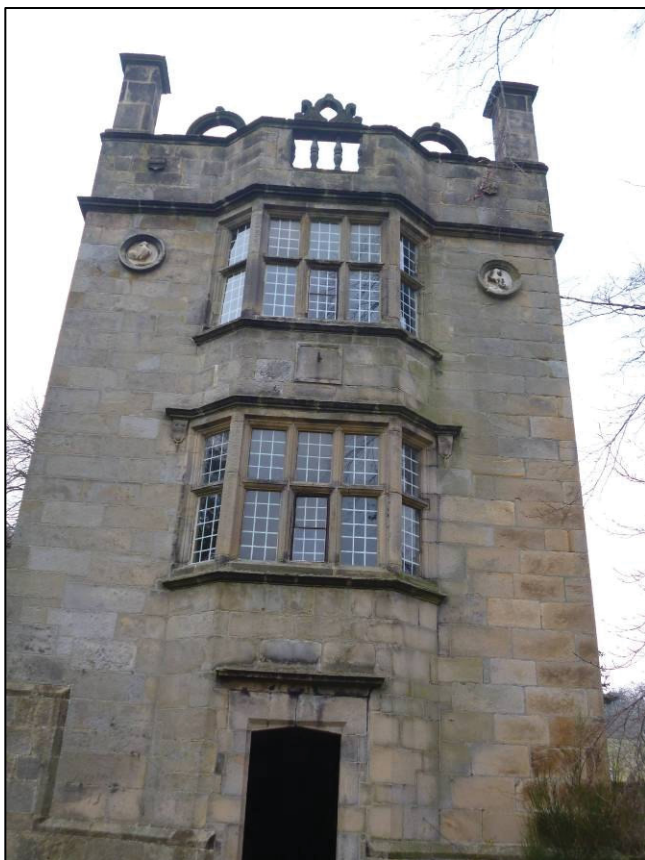
Plate 26: Weston Hall Banqueting House, south elevation, looking N.
