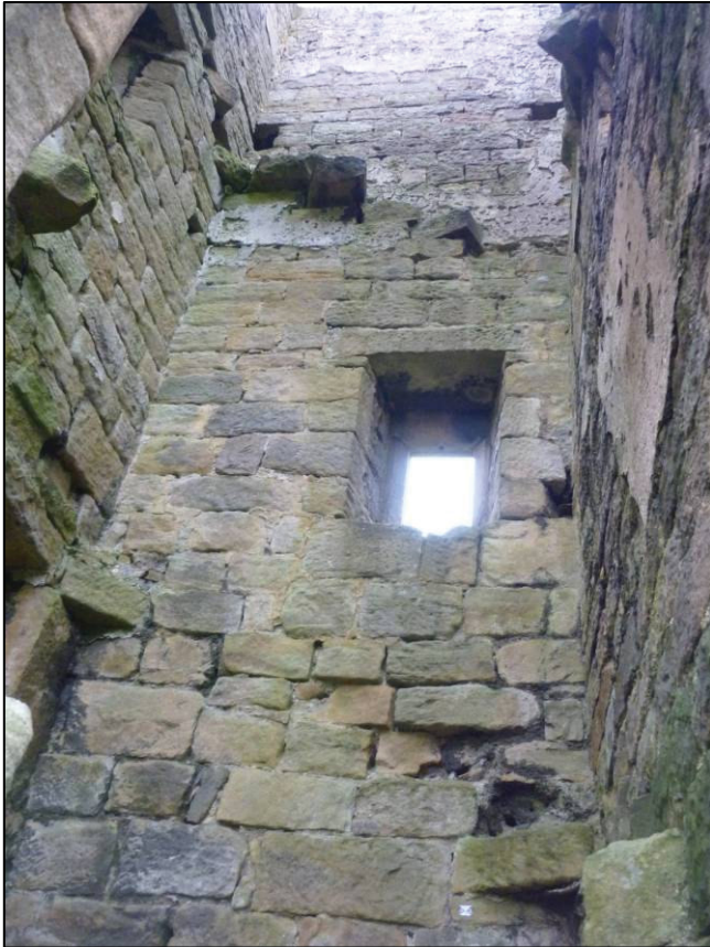
Plate 18: Internal north elevation of stair turret, looking N (photo 2/561).
