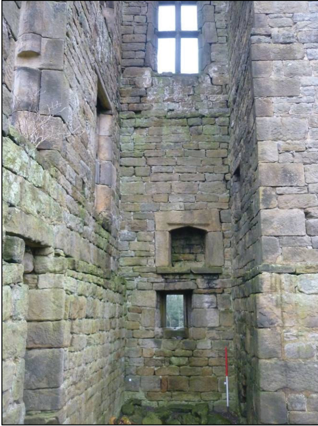
Plate 21: Elevation 25, looking NW (photo 2/539).
