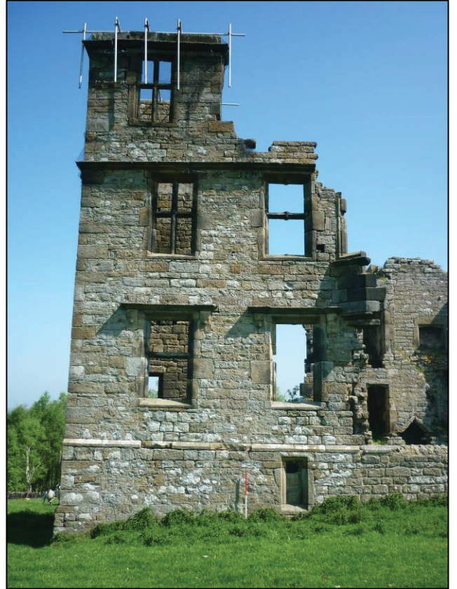
Plate 11: West end of elevation 11, looking NE (photo 3/204).
