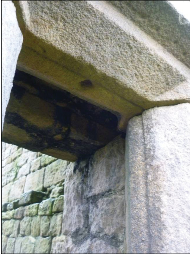
Plate 10: Window W10 in elevation 10, showing glazing slot etc (photo 2/534).
