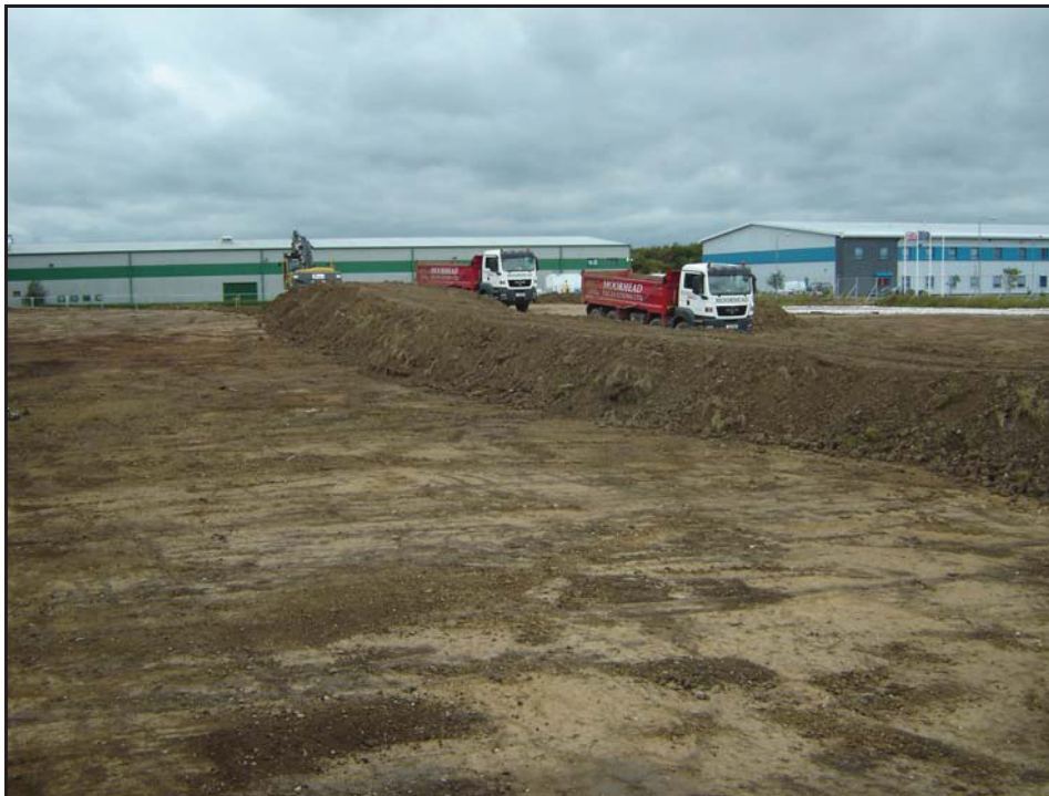
Plate 1. General shot of site during stripping, looking north-west
