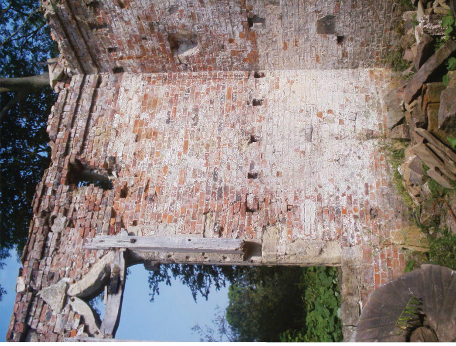
Plate 6. Interior of Howsham Mill (2004).
