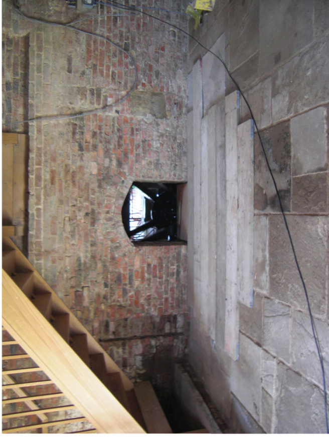
Plate 54. Howsham Mill Restored (May 2013).
