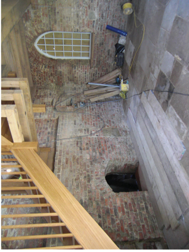
Plate 60. Howsham Mill Restored (May 2013).
