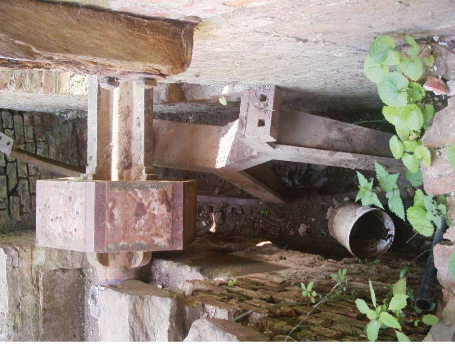
Plate 19. Interior of Howsham Mill (2004).
