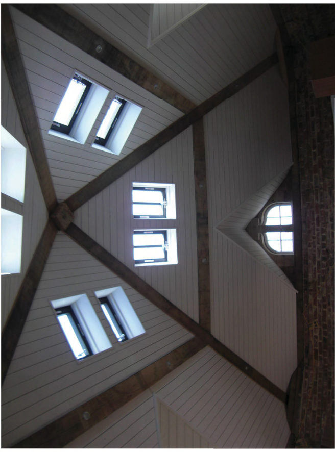
Plate 58. Howsham Mill Restored (May 2013).
