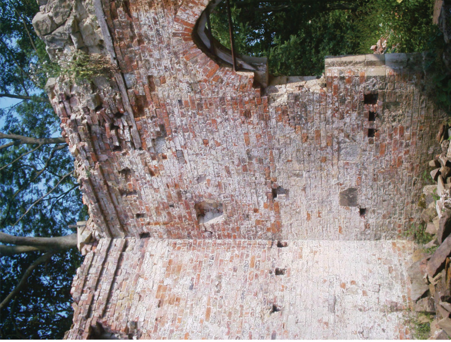
Plate 5. Interior of Howsham Mill (2004).
