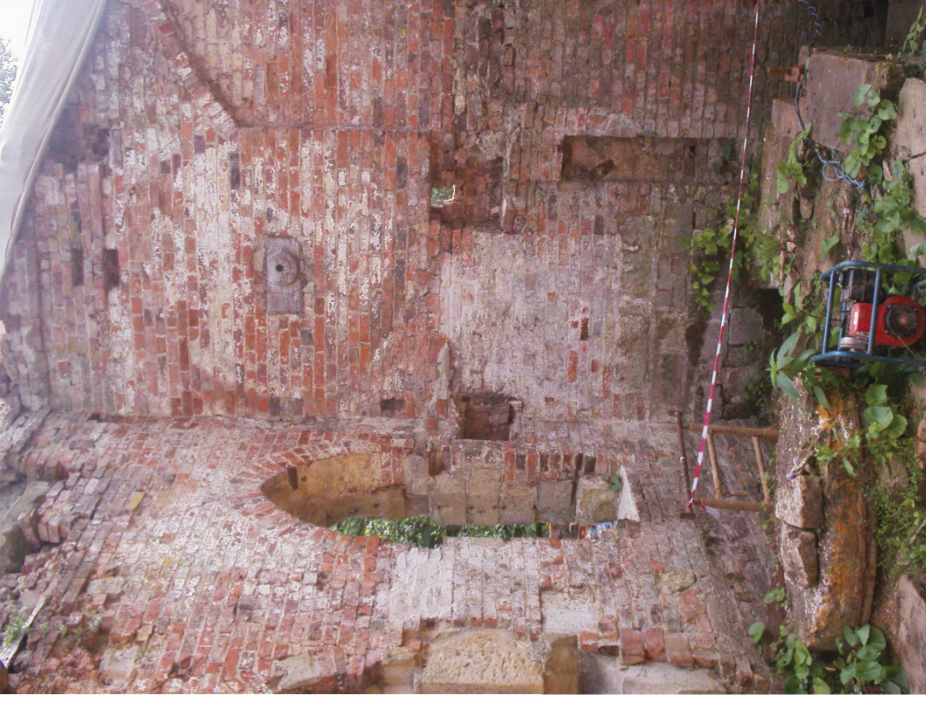
Plate 14. Interior of Howsham Mill (2004).
