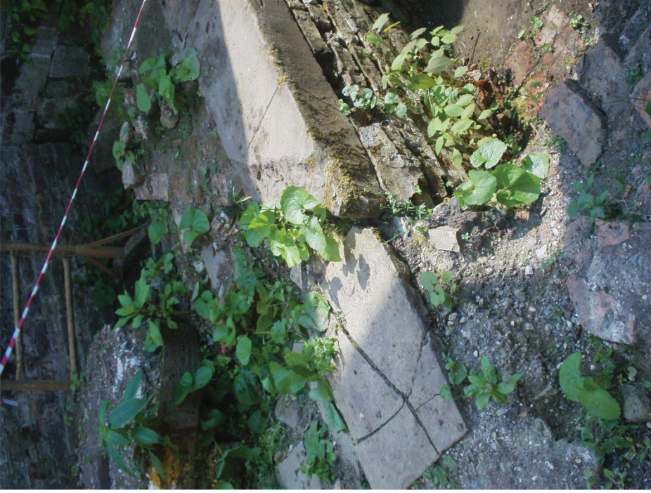
Plate 17. Interior of Howsham Mill (2004).
