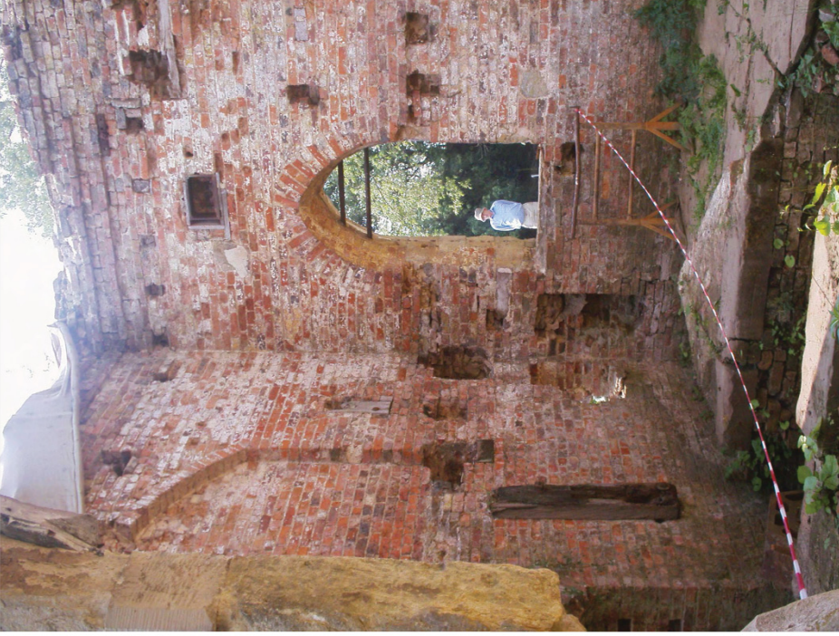
Plate 11. Interior of Howsham Mill (2004).
