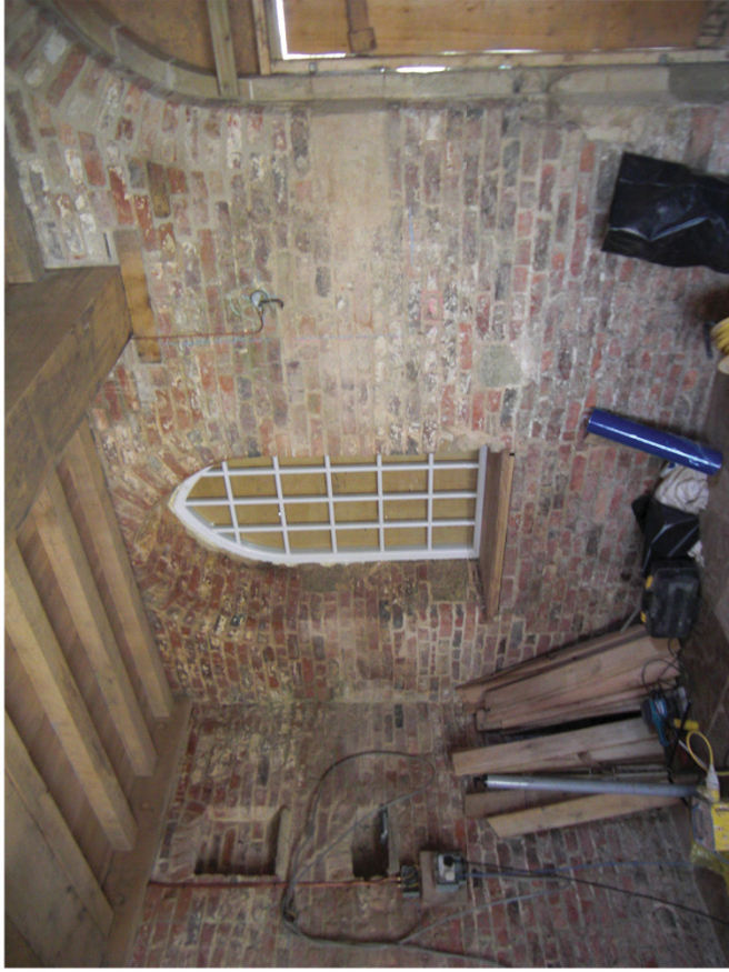
Plate 55. Howsham Mill Restored (May 2013).
