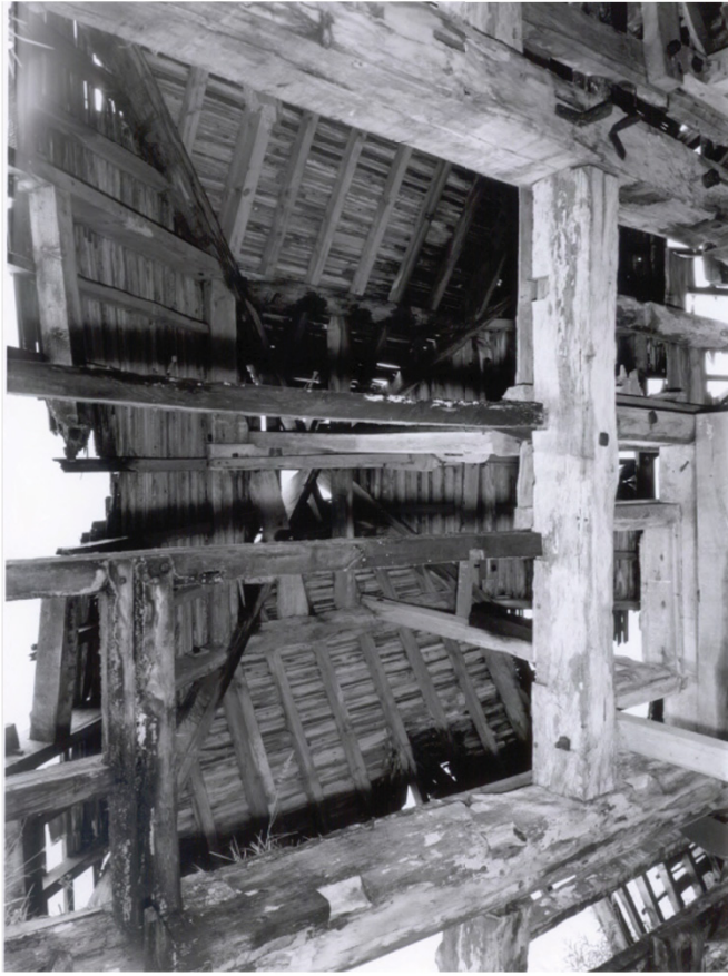
Plate 1. National Monument Record Shot of Howsham Mill.
