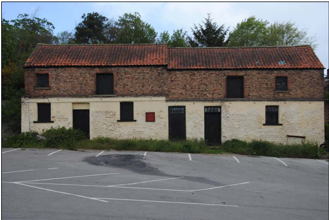
Figure 24: Former stable block, looking north
