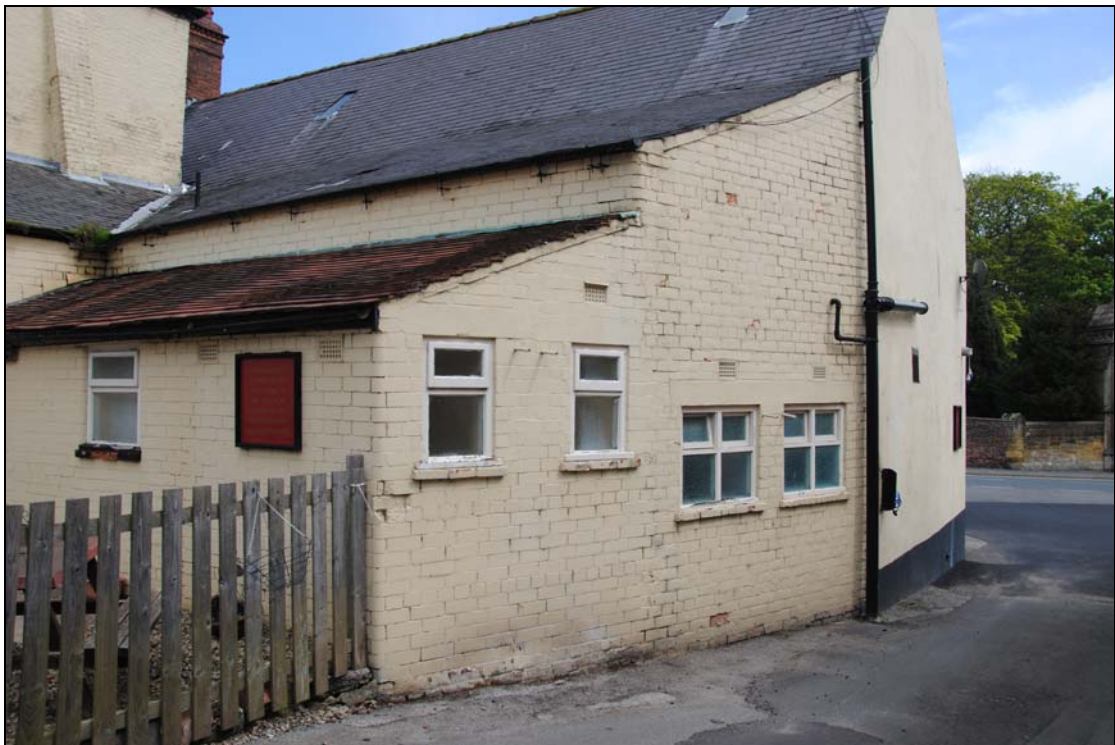
Figure 16: Toilet block added to rear of road frontage block
