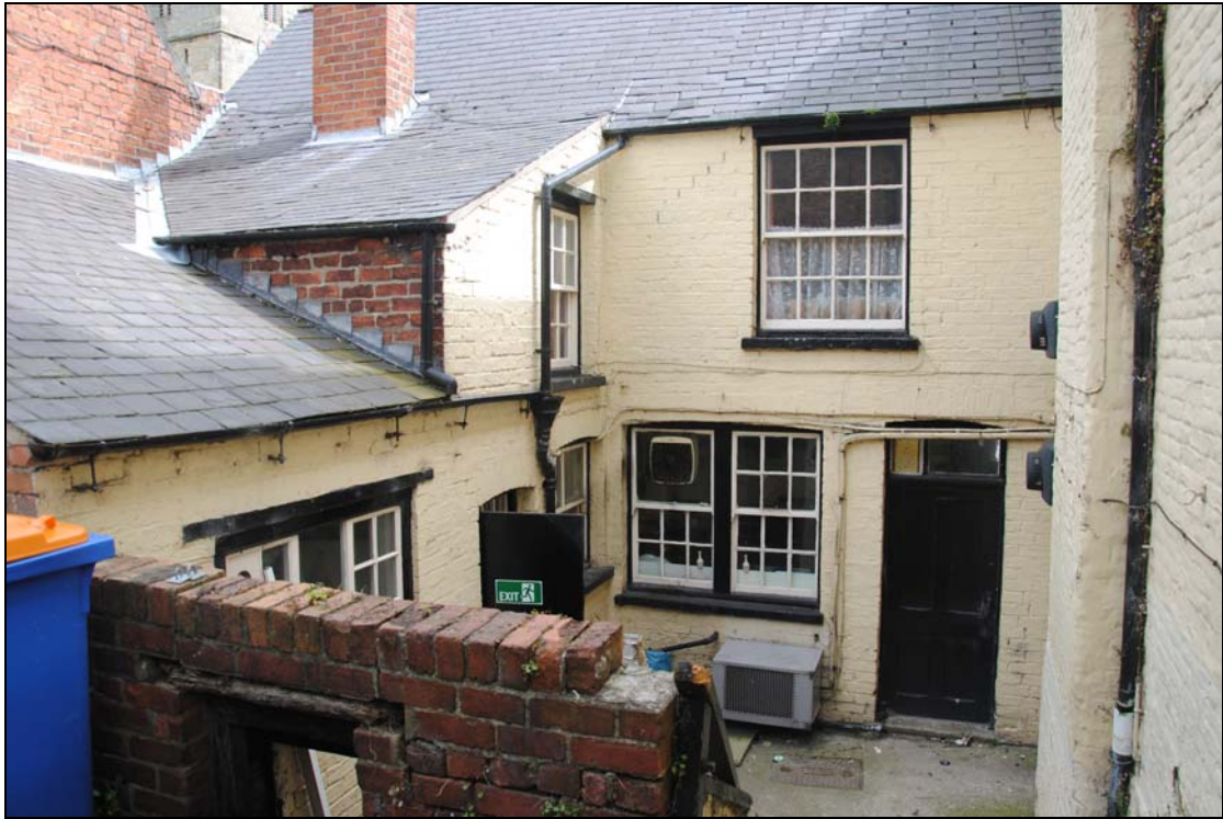
Figure 21: Domestic accommodation block looking east across internal yard
