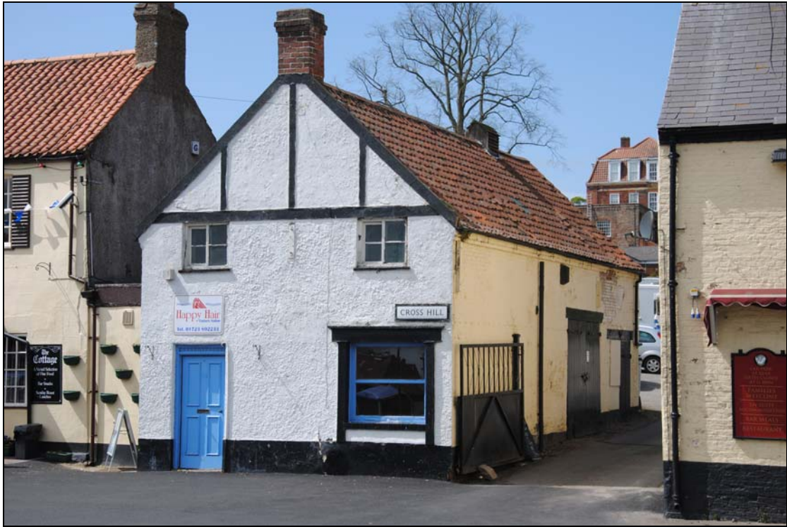
Figure 23: Former shop to south of car park entrance
