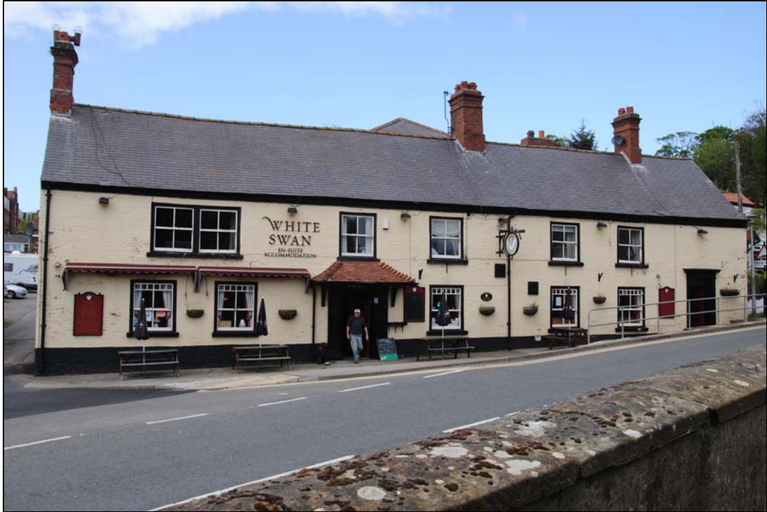
Figure 15: The road frontage block looking west
