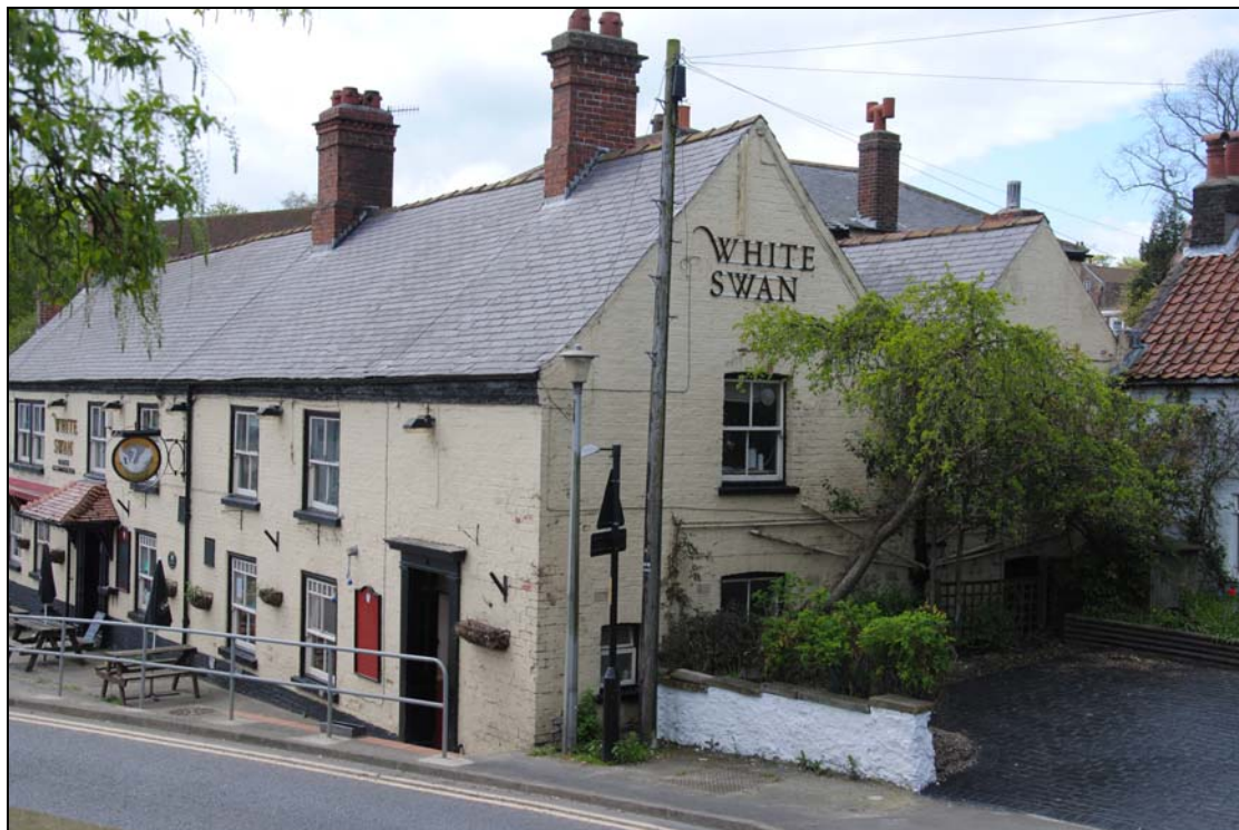
Figure 20: View from north east, showing roofs of domestic accommodation and clubroom
