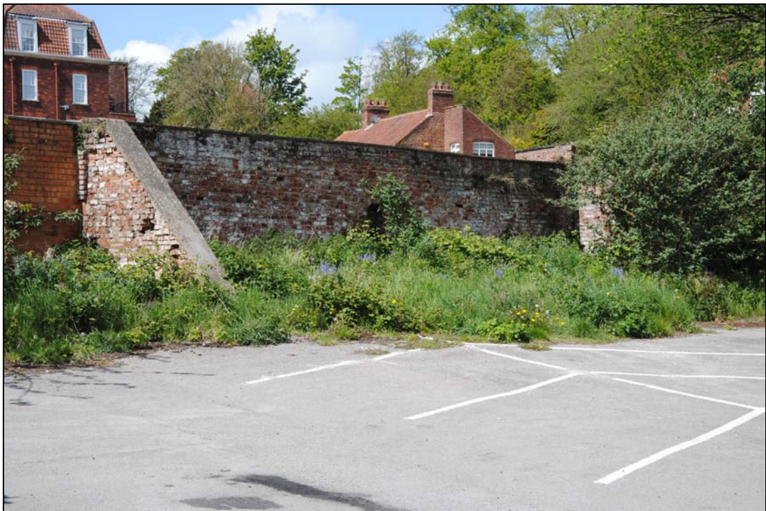
Figure 14: Old walls at west end of car park
