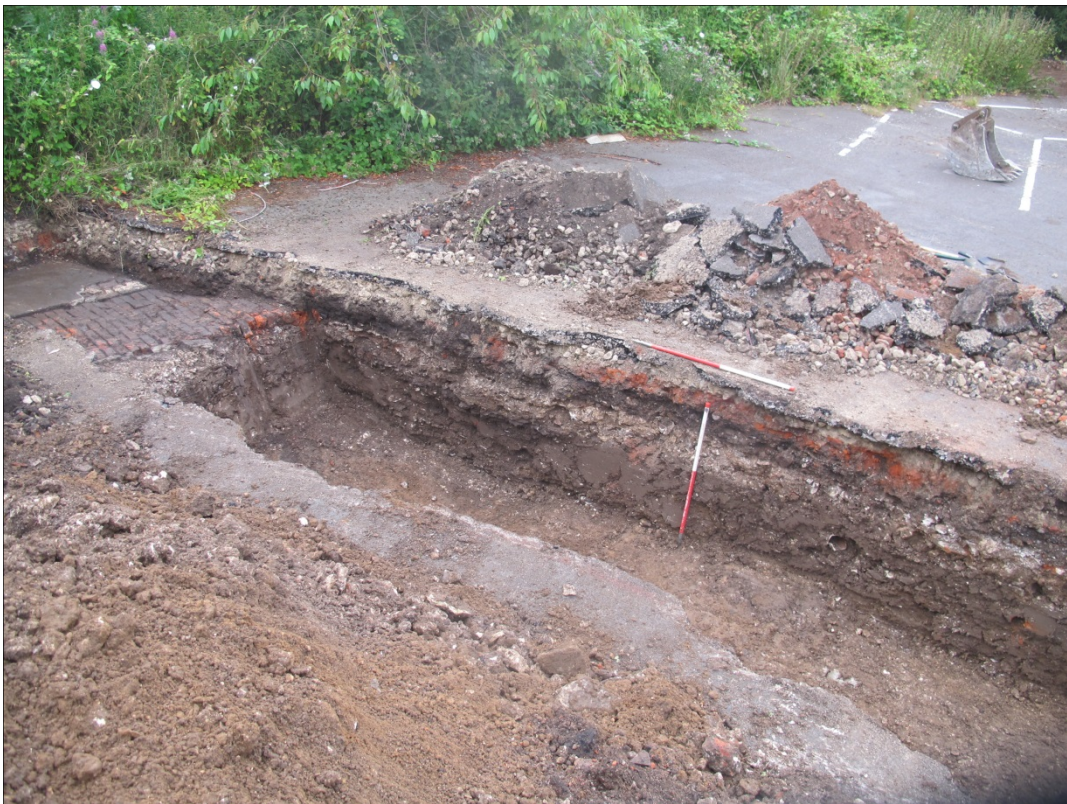
Figure 5: South-east facing section of Trench 1
