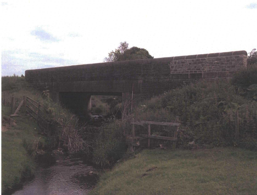
Plate 29: GBA12: Smallways new bridge
