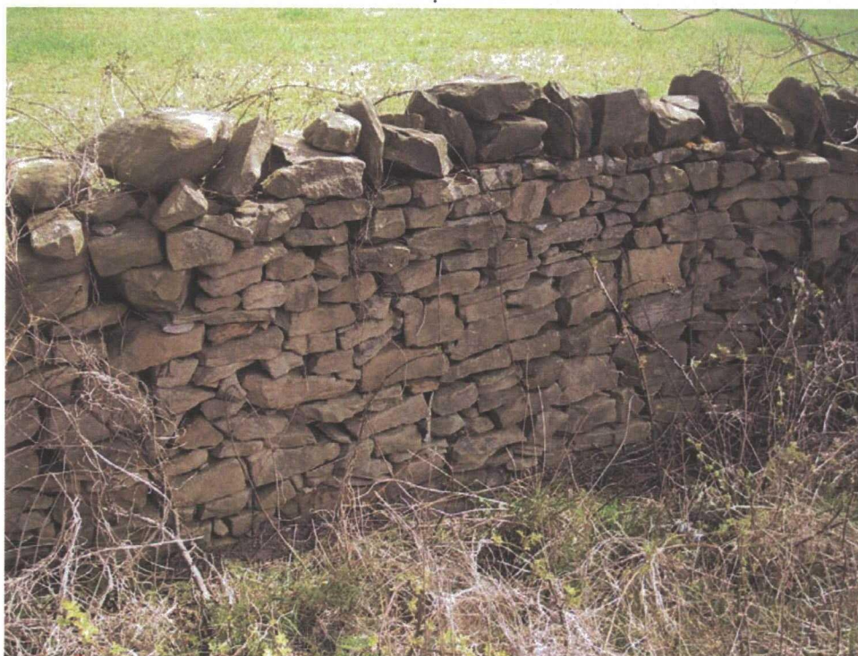
Plate 78: Site 015, showing details of the wall at the lay-by on Stephen Bank, to the south of the existing carriageway. Its construction is similar to that at Gatherley Moor Quarry. The wall has been extensively rebuilt in places
