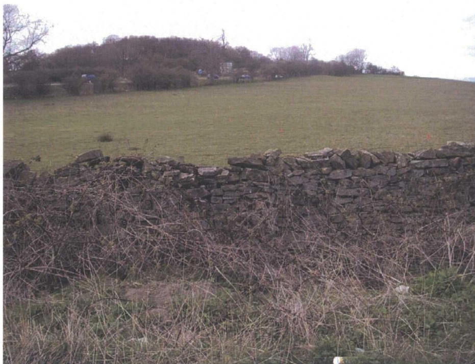
Plate 72: Site 009, field wall to the south of the carriageway taken on Forcett Lane, looking north-east. It appears to have been poorly rebuilt and shows signs of deterioration. Note the lack of quality in its construction compared to examples at Gatherley Moor Quarry
