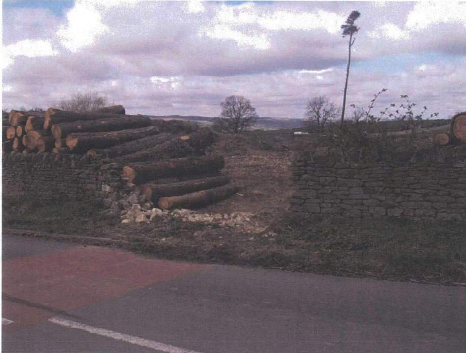
Plate 68: Site 005, western end of Gatherley Moor Quarry, taken from the north of the carriageway, looking north-west towards Carkin Moor. Note the removal of a substantial section of the wall at this location
