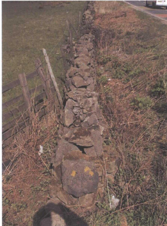
Plate 81: Site 018, wall at Carkin Moor, to the south of the carriageway, looking north-west. This displays evidence of stone removal and deterioration common to most of the field walls in the vicinity of the A66
