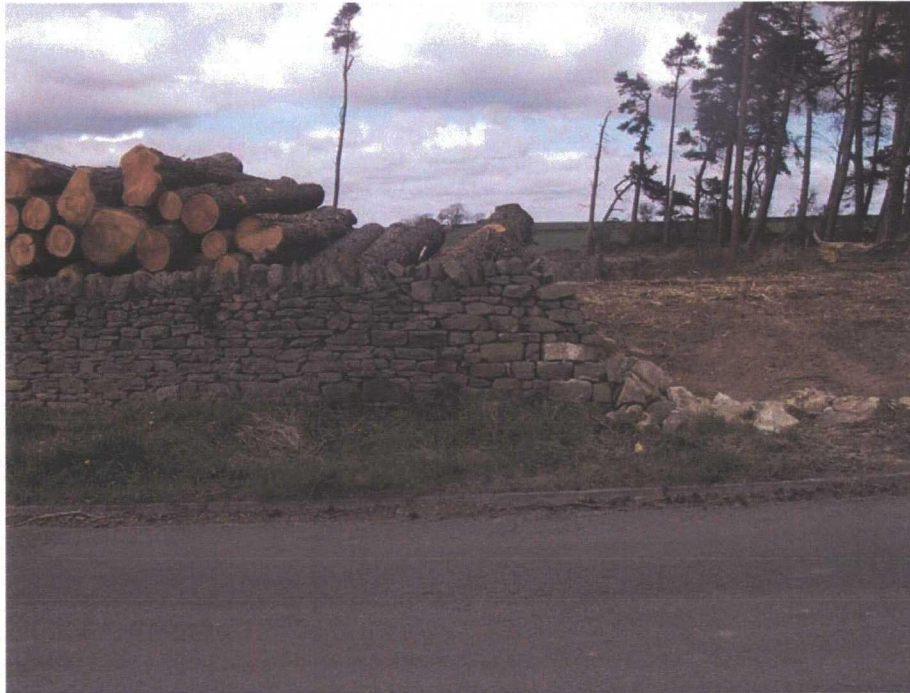
Plate 70: Site 007, western end of Gatherley Moor Quarry, taken from the north of the carriageway, looking north-west. Note the removal of a section of the wall at this location
