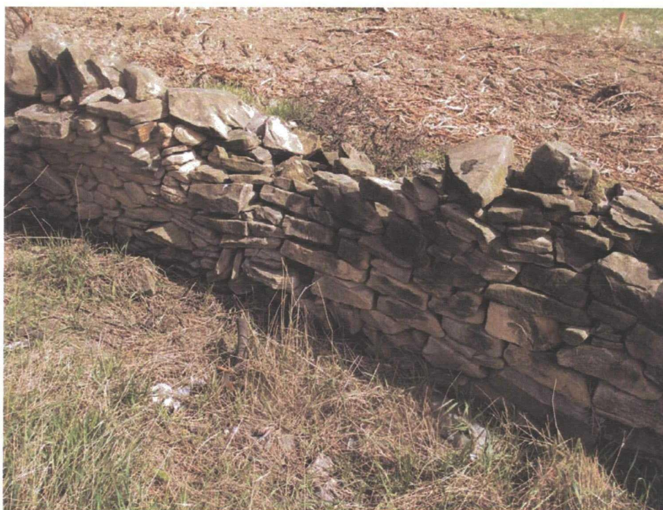
Plate 79: Site 016, showing details of the wall at the lay-by on Stephen Bank, to the south of the existing carriageway. Its construction is similar to that at Gatherley Moor Quarry. The wall has been extensively rebuilt in places, and has areas of collapse
