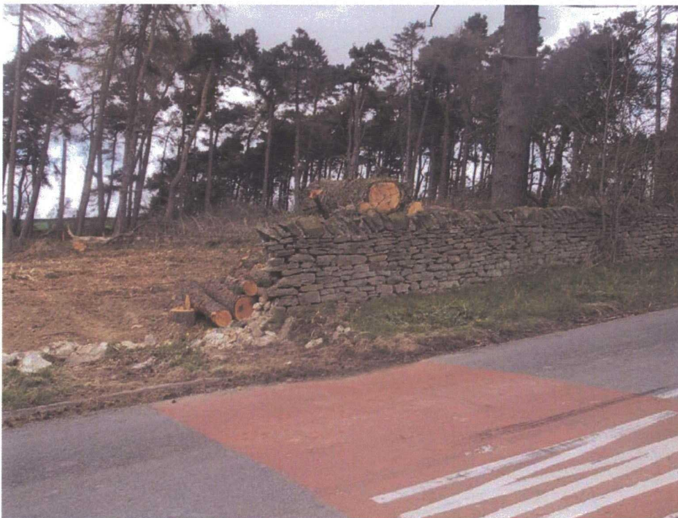
Plate 69: Site 006, western end of Gatherley Moor Quarry, taken from the north of the carriageway, looking north. Note the removal of a section of the wall at this location
