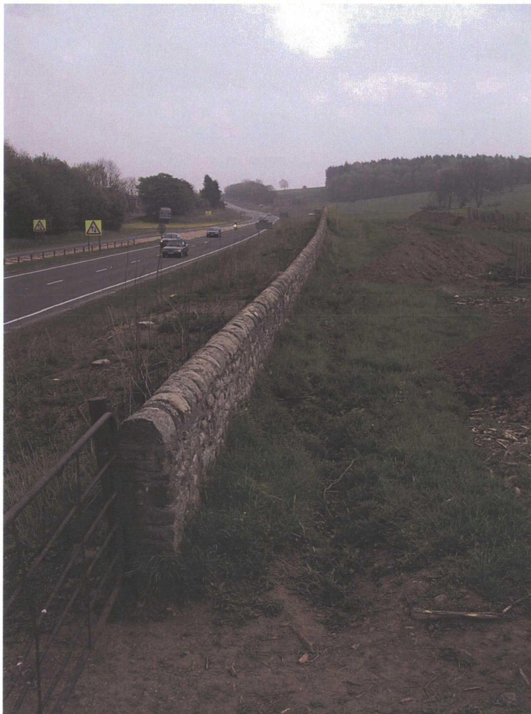
Plate 82: Site 019, wall opposite Thorpe Farm to the south of the carriageway, looking south-east. The wall is mortared and of a different style from the drystone walls, but of a similar style to the culvert headwalls, and is probably late twentieth-century in date
