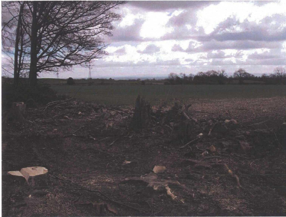
Plate 66: Site 003, the eastern end of Gatherley Moor Quarry, from the north of the carriageway, looking north. Substantial damage is evident and the majority of the wall does not survive
