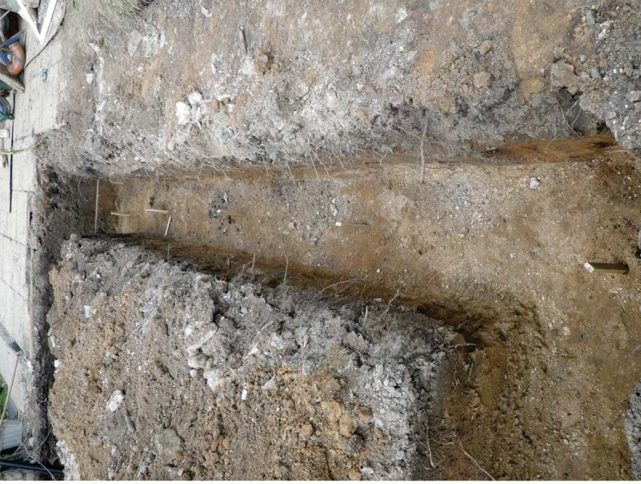
Plate 5. Strip Foundation Trench. Facing North.
