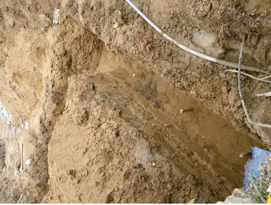
Plate 3. Strip Foundation Trench. Facing North-east.
