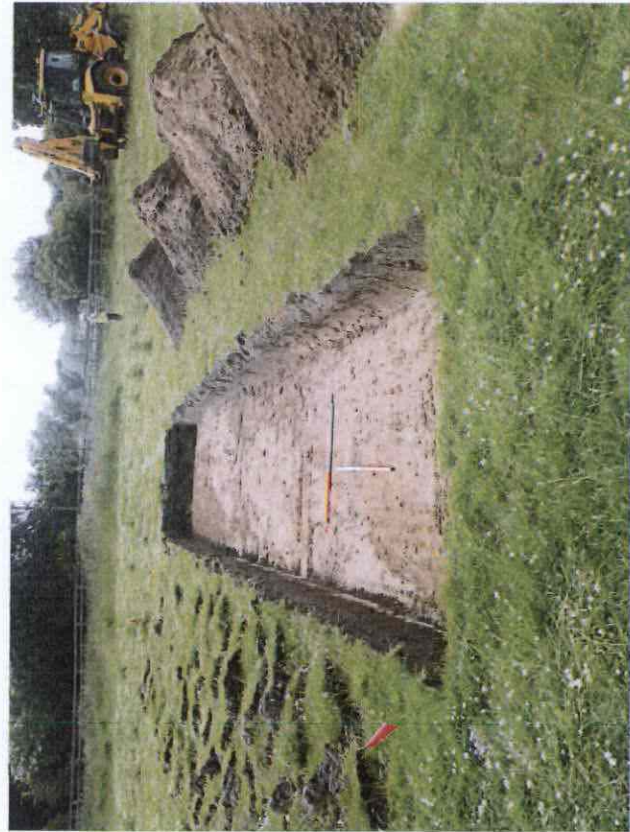
Plate 4. Evaluation Trench 1. Facing South.
