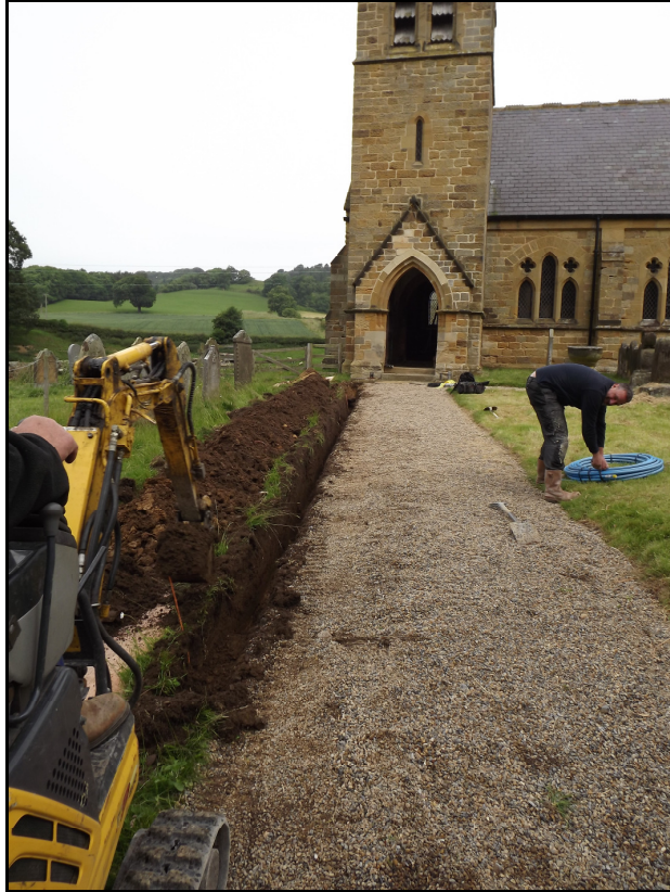
Plate 1. Cable trench under excavation, looking north
